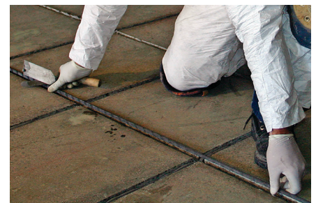
Near-Surface-Mounted FRP Reinforcement
