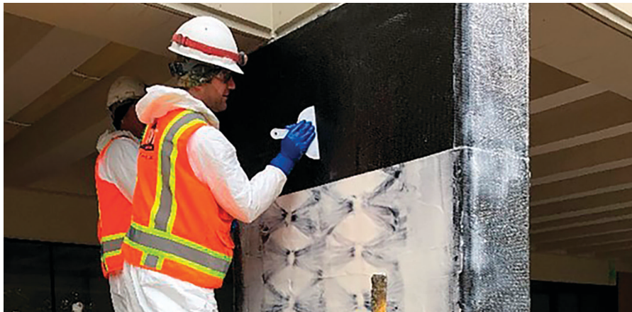
Large Aspect Ratio Column Confinement
