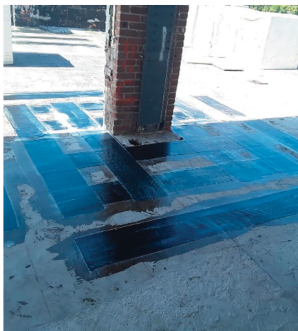
Slab Flexural Strengthening
