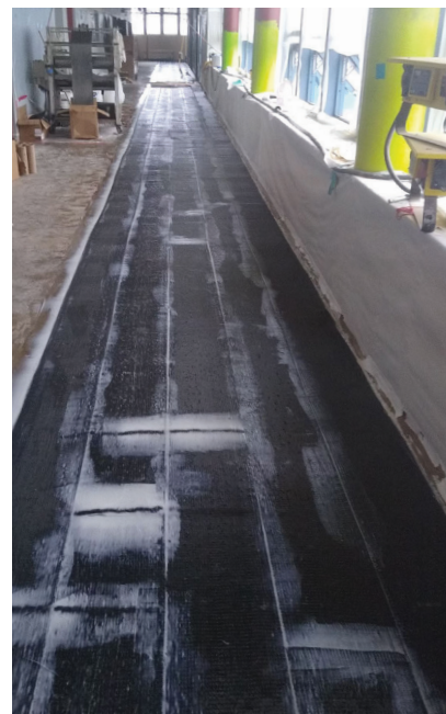
Collector Strengthening
