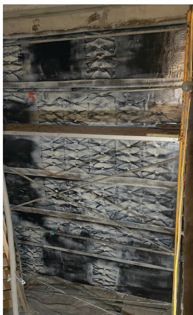
Wall Strengthening with FRP Anchors
