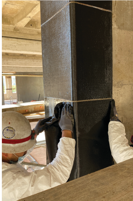
Boundary Element Confinement
