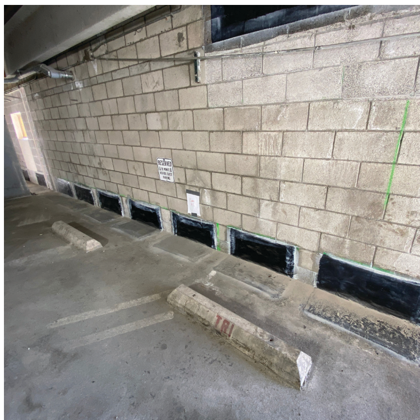
Slab-to-CMU Wall Joint Shear Strengthening
