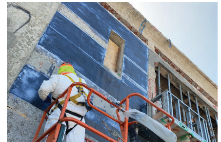
Shearwall Strengthening
