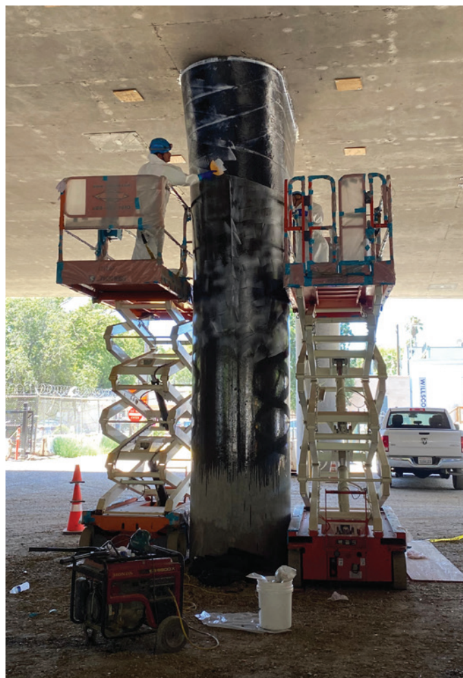
Fig. 4: Applied FRP jacket on the site
