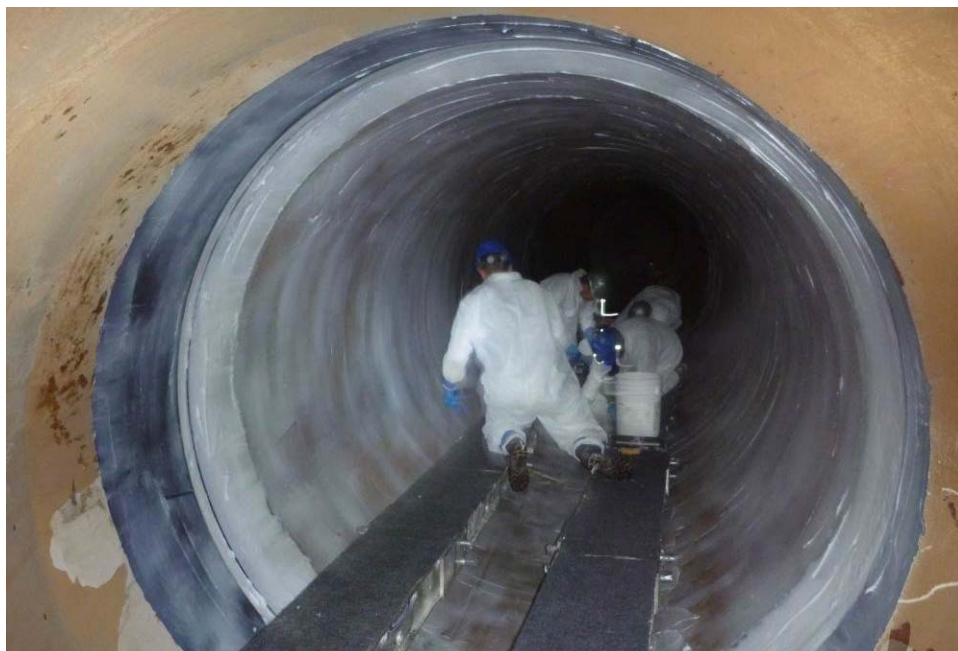
Figure 5. Installation of initial layer of thickened epoxy prior to installation of CFRP (Photo Credit: Hector Posada of Tucson Water)
