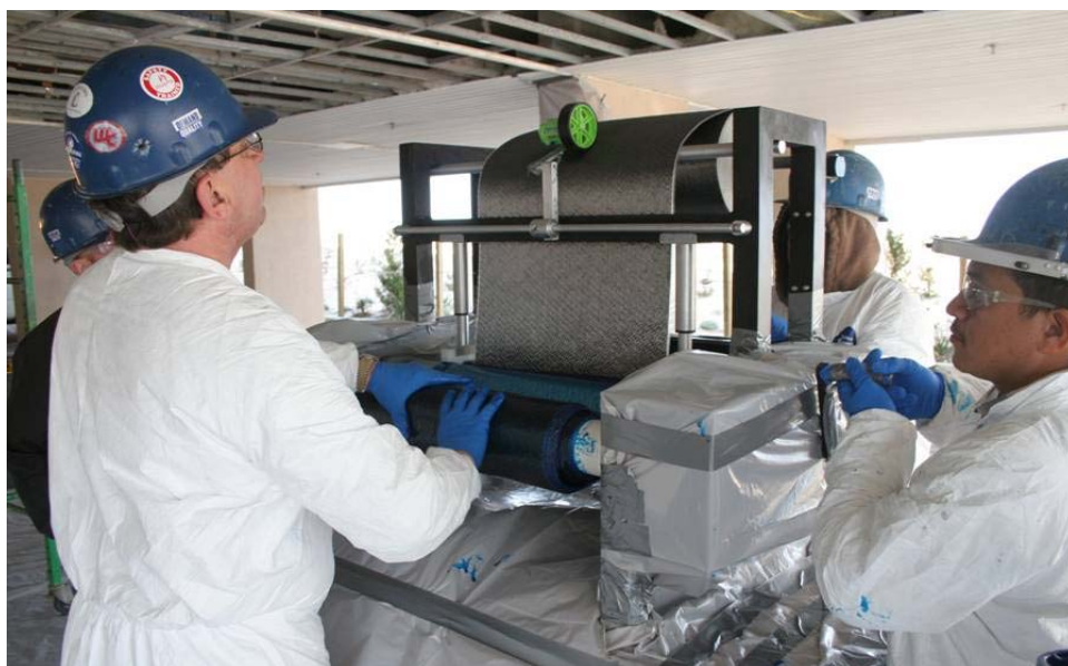
Figure 1. Mechanical saturation of carbon fiber fabric prior to installation in the pipeline
