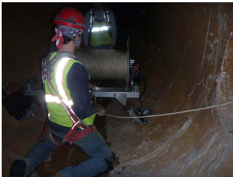
Figure 9. Re-installation of acoustic fiber optic cable after rehabilitation work was complete (Photo Credit: Hector Posada of Tucson Water)
