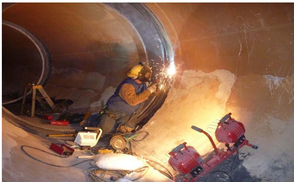
Figure 4. Welding of leaks in the joints prior to CFRP installation (Photo Credit: Hector Posada of Tucson Water)
