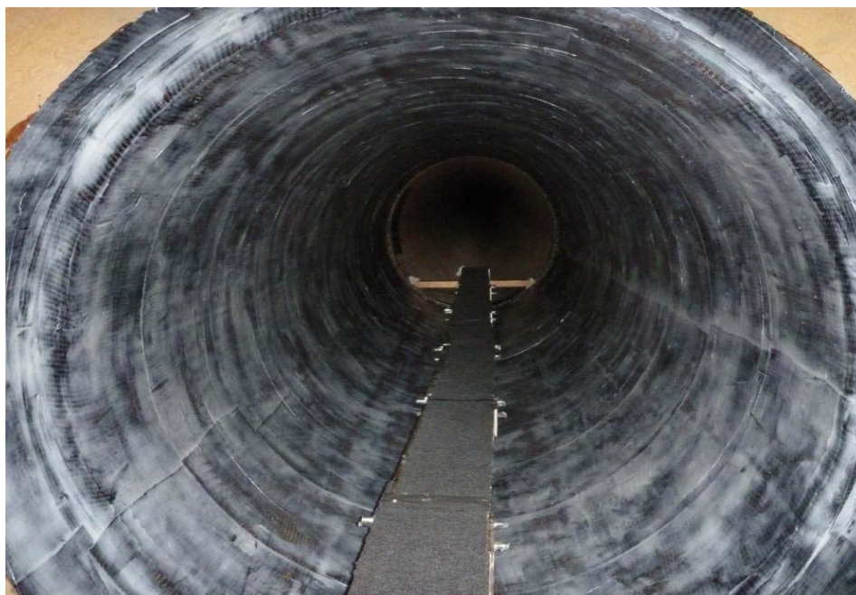
Figure 6. Completed CFRP lining (Photo Credit: Hector Posada of Tucson Water)
