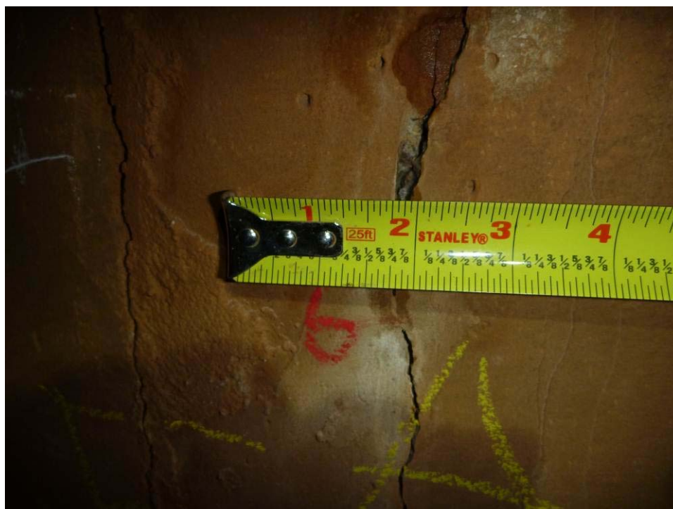
Figure 2. Observed joint damage (Photo Credit: Hector Posada of Tucson Water)
