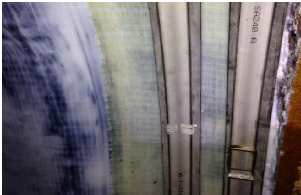
Figure 8. End termination Detailing
