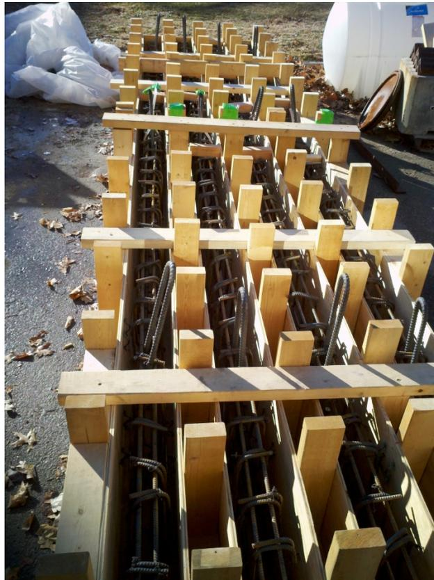
Figure 2—Caging inside of Formwork before Casting
