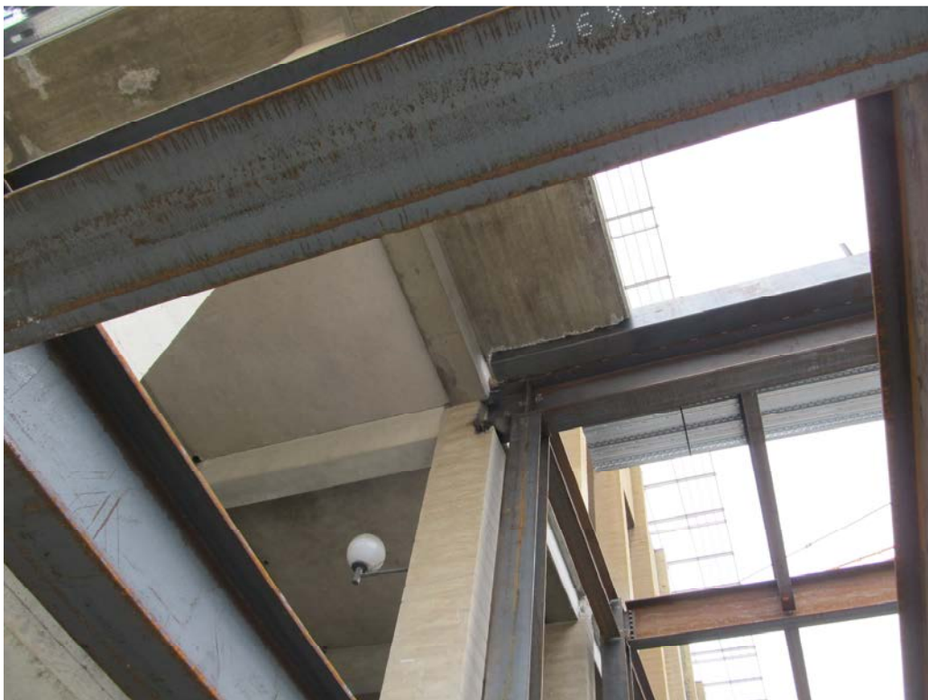
Figure 9- Connections between existing MLK diaphragms and new diaphragms of west addition designed based on forces calculated by PBSB methodology
