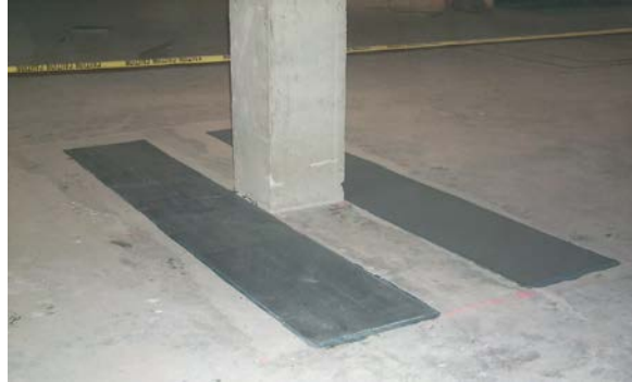
CFRP layout for negative moment strengthening
