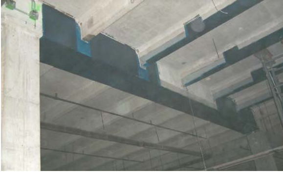
Strengthened beam and joists
