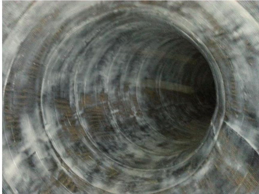
Figure 6. Completed CFRP installation
