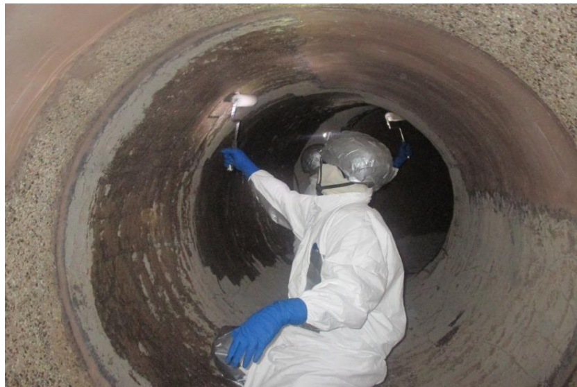
Figure 5. Primer epoxy being applied to concrete substrate of PCCP line
