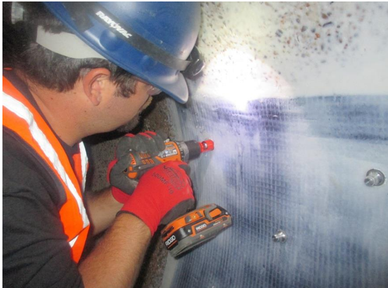
Figure 4. Preparation of test dollies for performing a pull test to verify surface preparation
