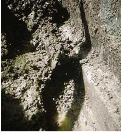
Figure 4. Without a filter to keep silt from contaminating the surrounding stone, drain tile can be rendered useless within just a few seasons (left). Pipe that is pre-wrapped or “socked” with filter material will prevent drain tile from becoming plugged (above). Various geotextiles are available in rolls, and pre-wrapped or “socked” pipe — pipe that is manufactured with a filter sleeve already in place — is also available.
