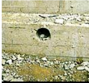
Figure 9a. An interior sump basket picks up excess water flowing through sleeves in the footing.
