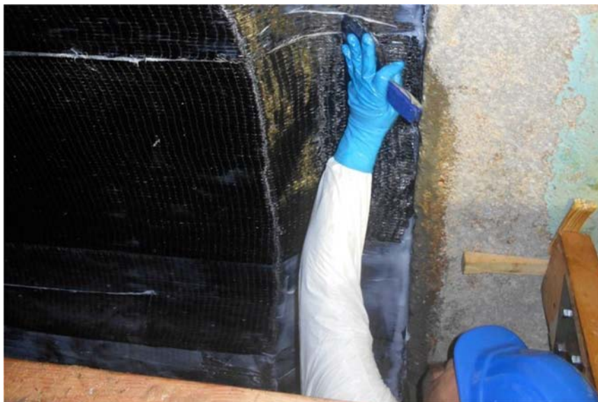
Figure 8. Completed termination detail
