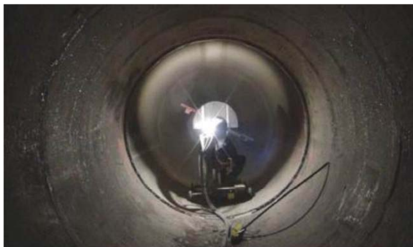
Figure 6. Sponge-blast set-up on pipe interior
