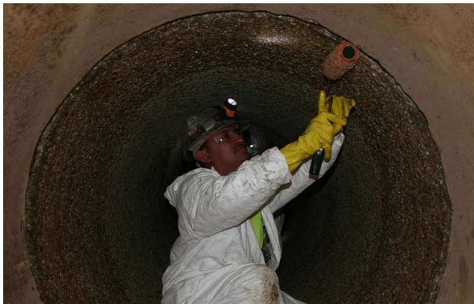
Figure 1. Application of epoxy primer
