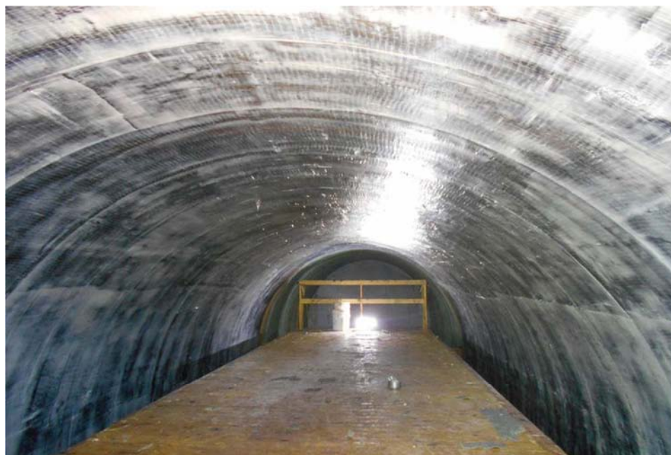
Figure 2. Completed CFRP lined section prior to removal of scaffolding
