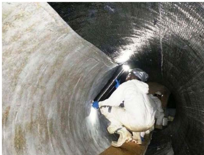
Figure 7. Installation of longitudinal layer of CFRP
