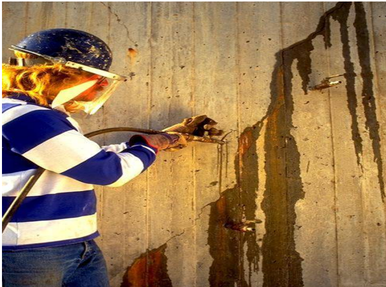
Figure No. 5 Following Port-to-Port Communication techniques, Chemical Grouting begins from the lowest to the highest injection port elevation.
