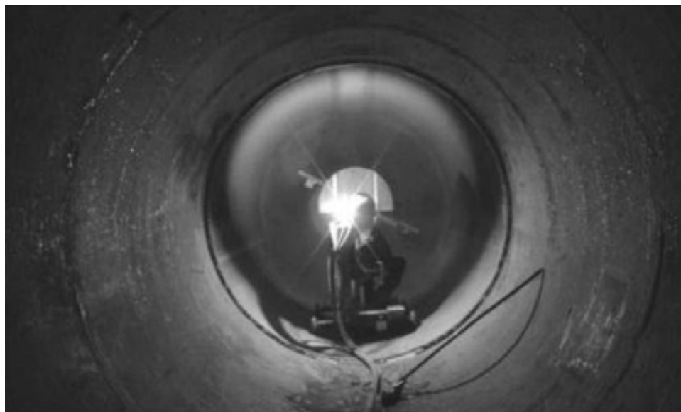
Figure 5. Sponge-blast set-up on pipe interior
