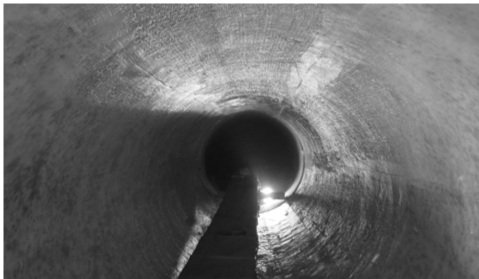
Figure 2. Installed longitudinal layer of FRP
