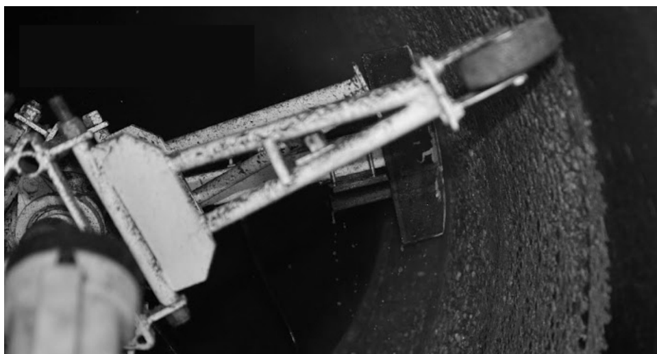
Figure 3. Surface preparation using water blasting equipment
