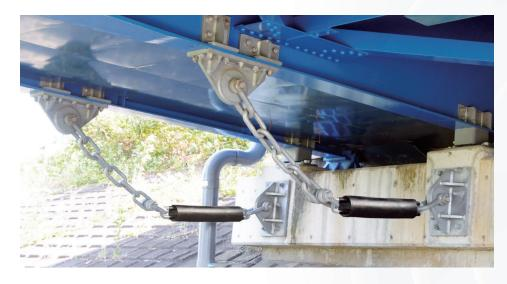
The Rubber Chain Restrainer System - Restraining Chain is a fail-safe system designed to prevent bridge unseating. It alleviates impact forces and accommodates transverse movements.
