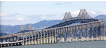
The Richmond San Rafael Bridge benefits from Lead Rubber Bearings as forces can be redistributed throughout the structure. Without the Lead Rubber Bearing, the significant height differences of the piers would cause the shorter, stiffer piers to attract the majority of the lateral force. The structure required a higher than normal level of initial strength because of high wind loads.
