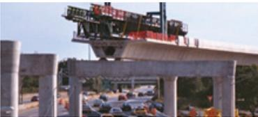
The elevated JFK Light Rail System connects JFK Airport to the New York subway system. The bridge is 10 miles long and is supported by 1,364 DIS isolators. The design-build contractor chose isolation to save on foundation costs. As the foundations were smaller, significant other cost savings were realized by minimizing the relocation of underground services at the airport and along the Van Wyck Freeway.
