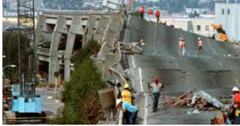
Conventionally designed structures rely on an inelastic response in select structural elements to dissipate earthquake energy, which results in permanent damage to the structure. STRUCTURAL TECHNOLOGIES offers an alternative design approach that incorporates isolation technology to safeguard the structure against the devastating effects of an earthquake.
