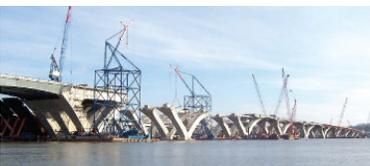
Woodrow Wilson Bridge spans the Potomac River near Washington, DC. This critical bridge, which carries over 250,000 vehicles each day, is in a low seismic zone. However, the redistribution of forces and performance under service-load conditions made seismic isolation an appealing option for the designers.
