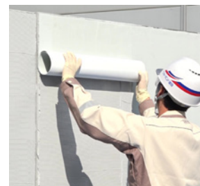
Install SHO-BOND Hybrid Sheet
