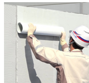
Install SHO-BOND Hybrid Sheet
