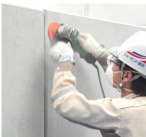
Remove weak parts and clean
