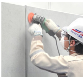
Remove weak parts and clean
