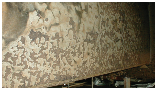
Figure 4 – Soot-stained concrete surfaces don’t necessarily mean that the concrete surfaces exposed to a fire are “fire-affected” to a point requiring repair.
