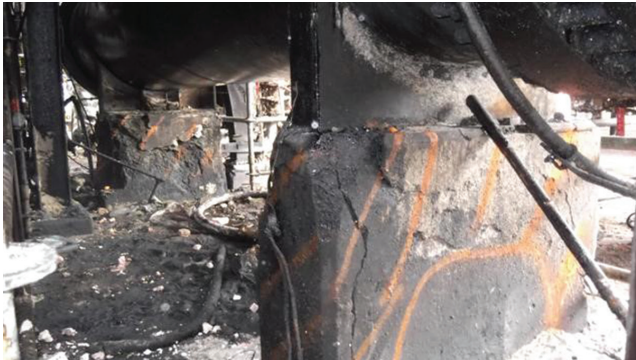
Figure 1 – Heat Exchanger Foundations exposed to a long duration Hydrocarbon-fueled fire event creating concrete delaminations (i.e., partially detached near surface internal separations) and spalls (i.e., detached delaminations), exposing embedded reinforcing steel and anchor bolts.
