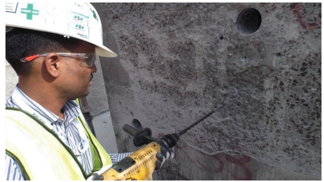
Figure 8 – Drill Probe performed adjacent to core sample location that's used to determine the extent & depth of concrete damage excavation is a quick accurate method of determining repair parameters.
