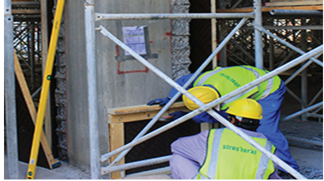
Figure 11 – Fire Damage Concrete Repair QA/QC Control Document providing a verifiable audit trail on-site requiring Hold Points, Witnessing and Sign-Off prior to proceeding with repair activity “milestones”.
