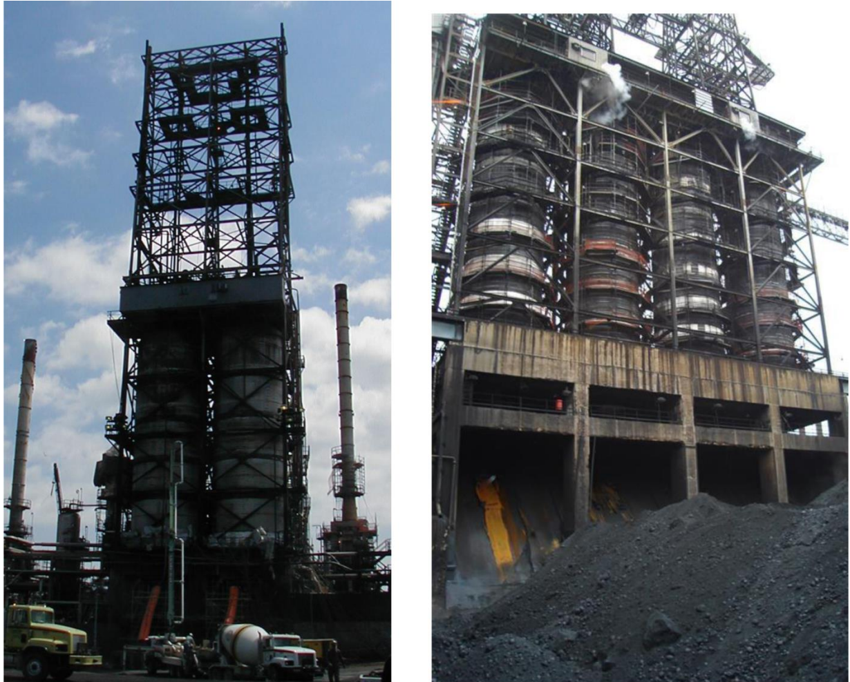
Figure 1 - Delayed Coking Units - Courtesy of Structural Group, Inc.
