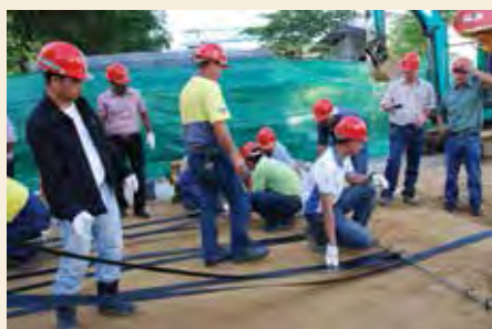
Installing polymeric VSoL® strips.
