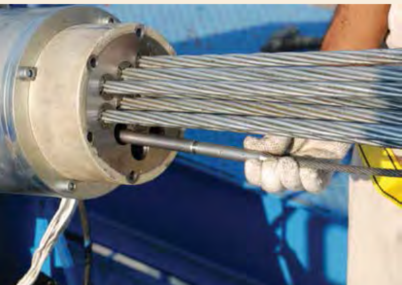
Strand installation during Stay Cable training.
