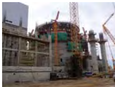
The LAES nuclear power project in Russia required VSL to provide an extensive monitoring system for the two reactor containments. Particular innovations in the project include the use of optical Bragg sensors to allow measurement of concrete deformation and temperature along post-tensioned tendons.
