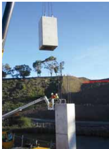
VSL's first precast pier project in 2007: Erection of precast pier segments at the remote Moorabool Bridge site in Geelong, Victoria.
