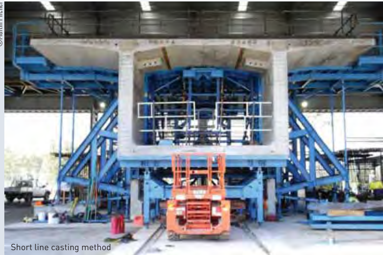
Short line casting method
