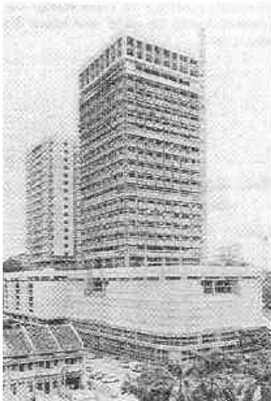
Figure 68: The Orchard Towers shortly before completion
