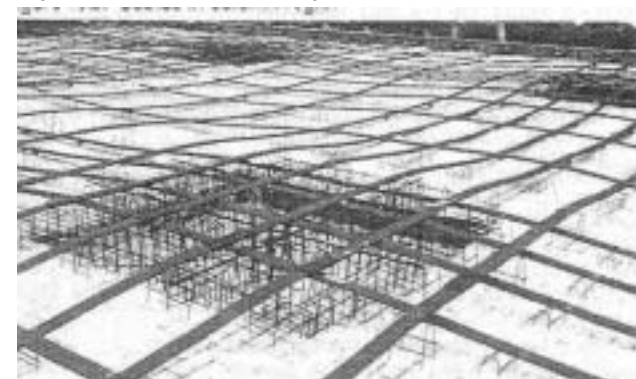
Figure 102: Cables in column region
