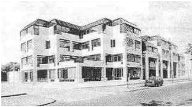
Figure 89: The finished Municipal Construction Office Building
