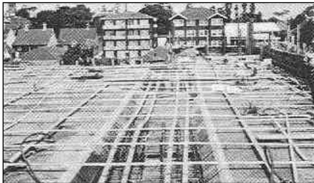
Figure 87: Positioned cables
