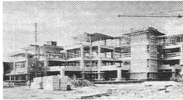
Figure 91: The building during construction
