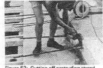
Figure 52: Cutting off protruding strand lengths
