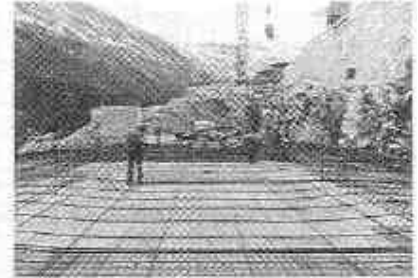
Figure 48: Supporting of tendons
