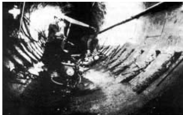
Prestressed concrete lining as an additional lining for the 11.4 km long pressure tunnel of the Piastra-Andonno hydroelectric power plant in Italy.
