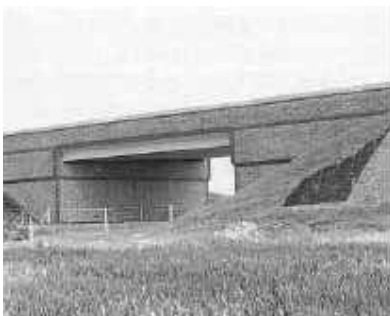
e) Glinton-Northborough Bypass, [4], Courtesy of Cambridgeshire County Council and Armitage Brick Limited
