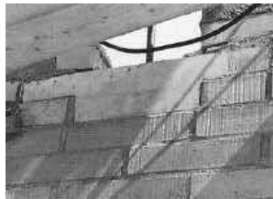
d) Placement of precast element
