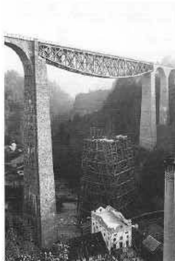
c) Railway Viaduct, Switzerland
