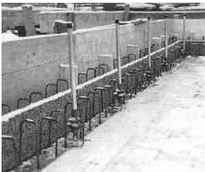
a) Placing of dead-end anchorages
