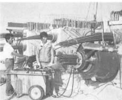
Figure 33: Stressing a VSL tendon
