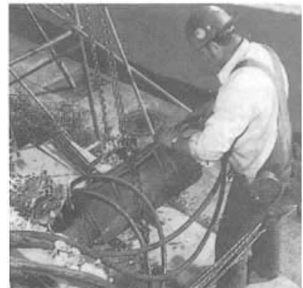
Figure 66: Stressing added tendons
