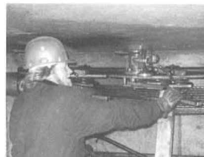
Figure 58: Pushing trough strands
