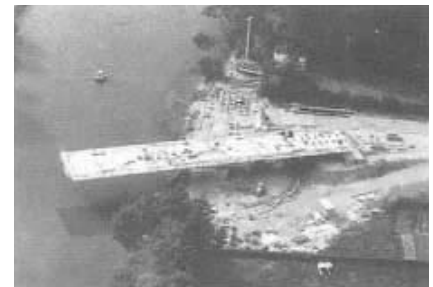
Figure 46: One bridge half nearly completely rotated
