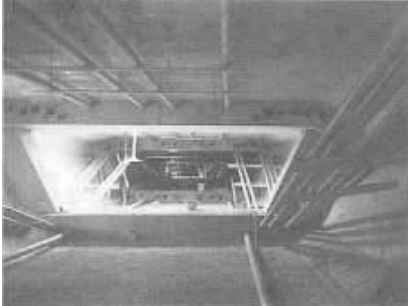
Figure 50: Tendons inside the box
