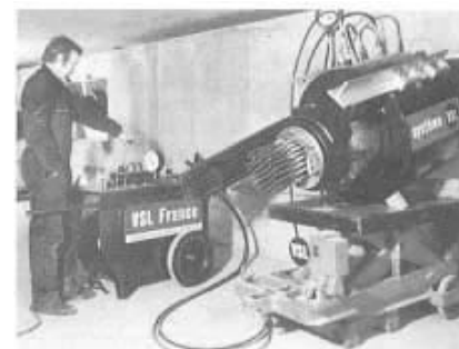
Figure 59: Stressing of additional tendons in the stressing chamber
