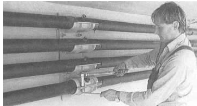
Figure 30: Intermediate tendon supports
