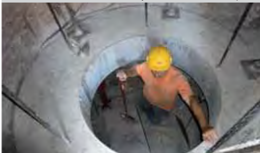
An intermediate ring was fitted.
