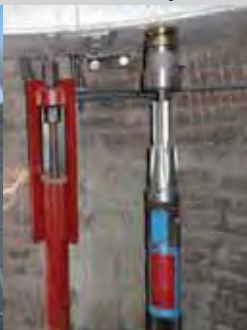
The first-stage stressing operation used a low-capacity jack.
