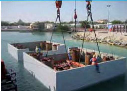
Setting a precast shell over the piles
