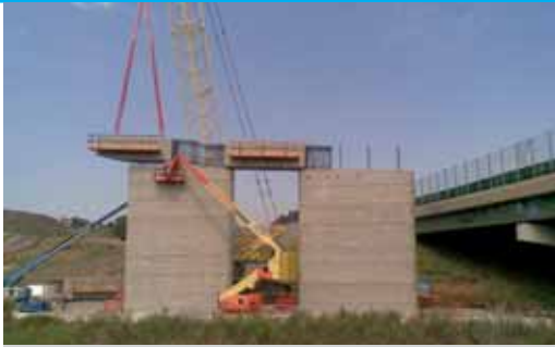
Placement of a crosshead unit on match-cast pier columns
