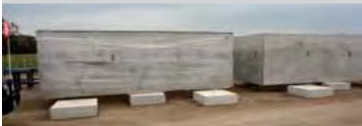
Match-cast pier segments in storage
