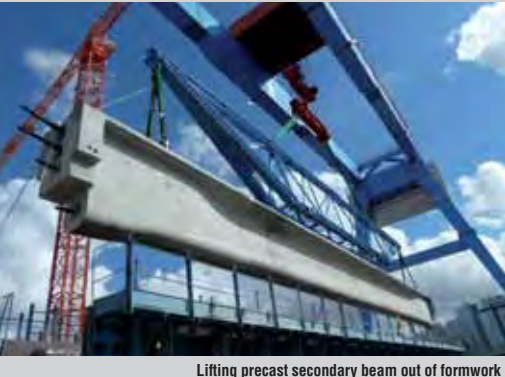
Lifting precast secondary beam out of formwork
