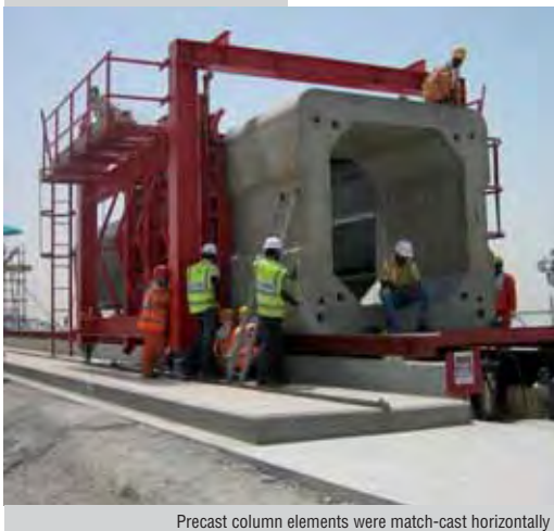
Precast column elements were match-cast horizontally
