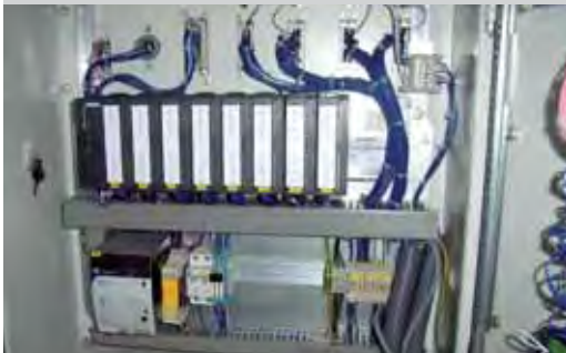
The heart of the control desk with a programmable logic controller (PLC)
