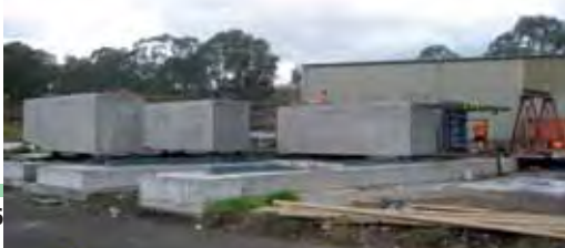
Precast crosshead segments
