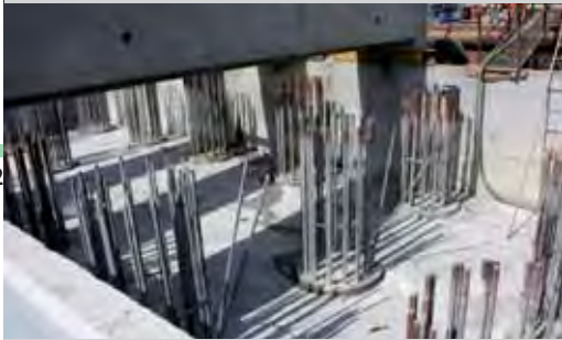
A precast shell, ready for setting steel reinforcement
