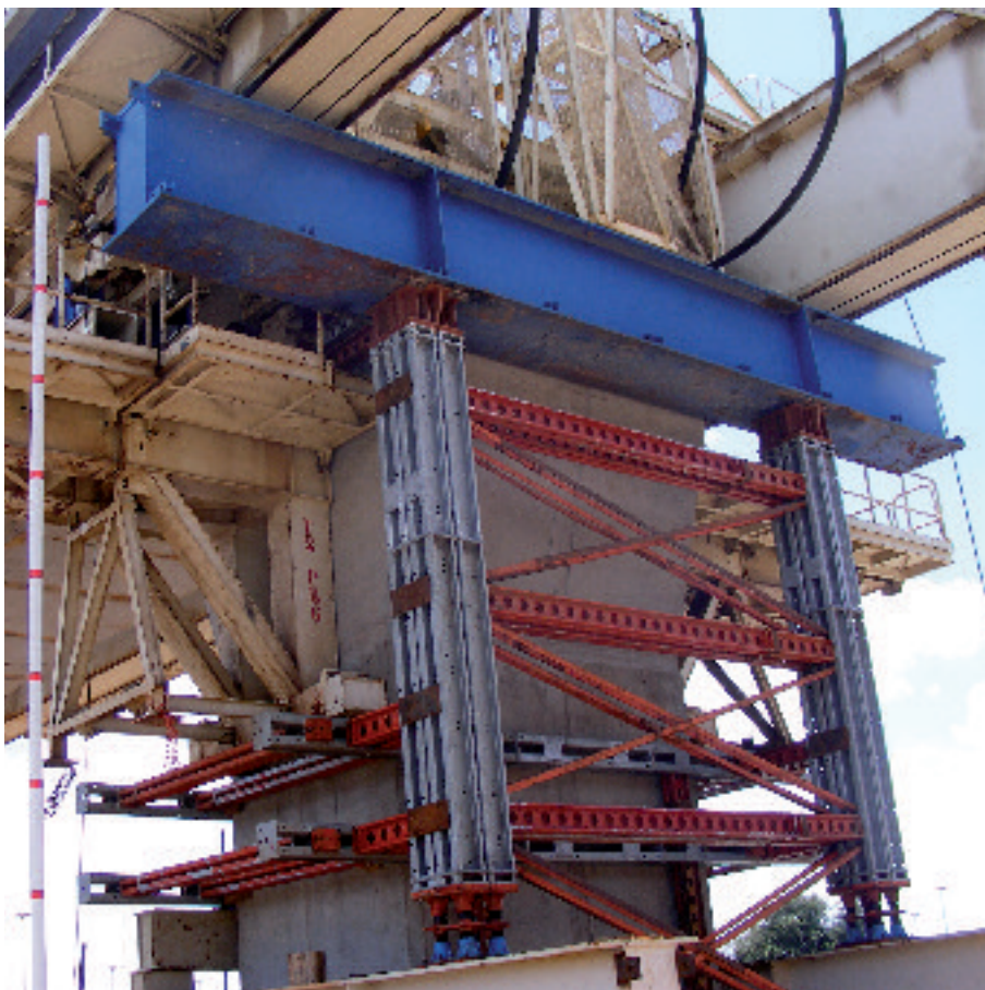
Temporary propping: 28 spans propped; 3,000m of stress bars supplied by VSL in Melbourne; 450t capacity per prop column.
