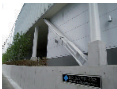
Sumitomo Rubber Industries Technical Centre in Kobe, Japan, equipped with brace damper.
