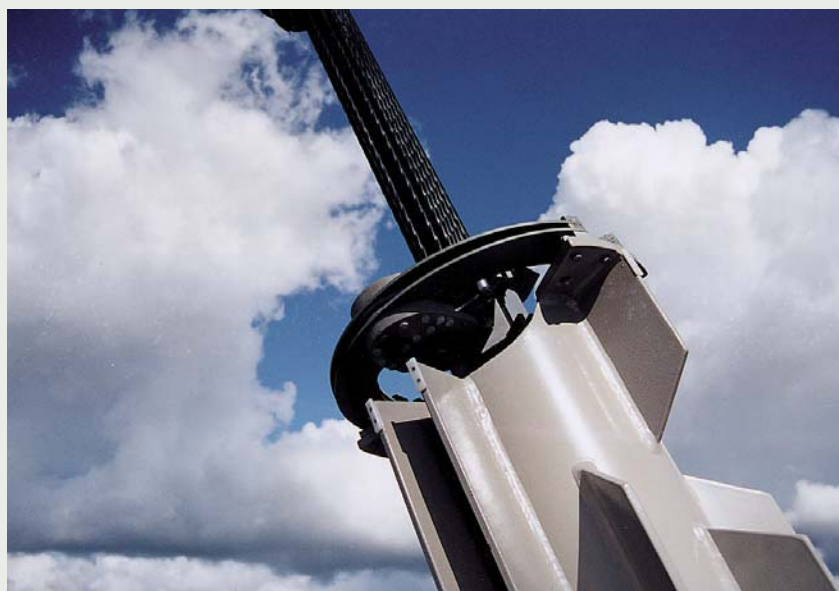
VSL Friction Damper on Uddevalla Bridge, Sweden
