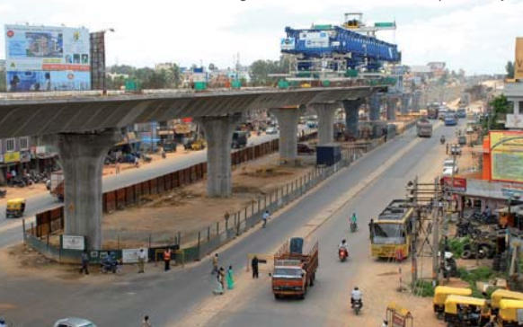
Bangalore - Hosur Elevated Expressway
