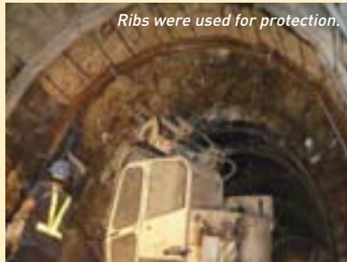
Vault cutting took place before the each section of demolition.
