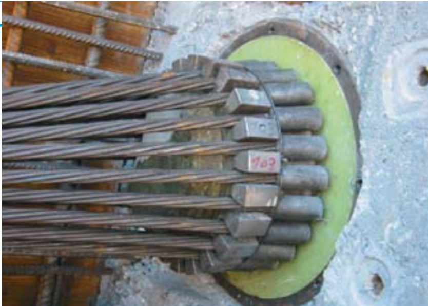
Plastic caps complement the encapsulation over the anchor head. The CS 2000 bearing plate was designed as a composite plate made of ductile iron and high performance mortar.
