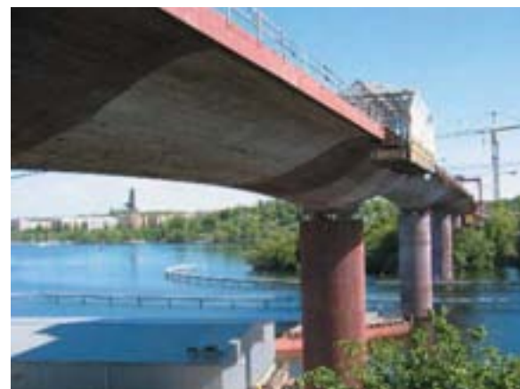
Electrically-isolated tendons have been used on this rail bridge in Sweden to minimise the risk of stray currents.
