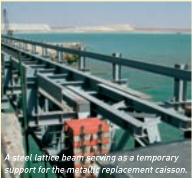
Beam fitted with 12 SMU 40 jacks and full-scale hydraulic launching and sliding system.
