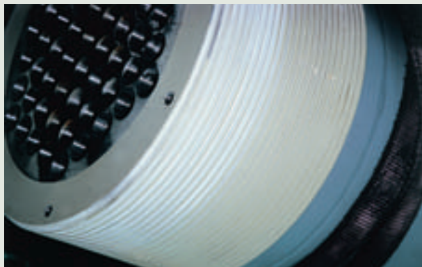
Anchorage protected by aluminium metal spraying.
