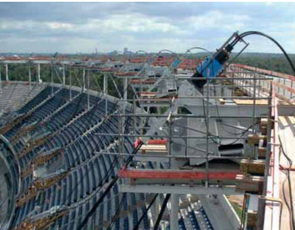
The total pulling capacity of the 88 units exceeded 21,000 t.
