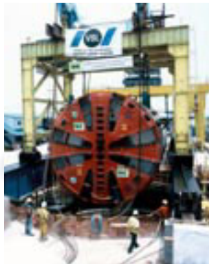
Tunnel Boring Machine, Singapore
