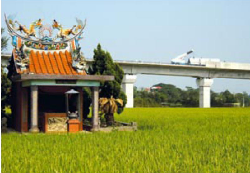
12 Long distance travelling. The girders travel up to 20 kms from the point of casting.
