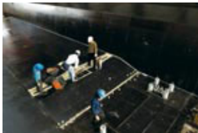
2 Preparation of the mould. Formwork (square frame with a few transverse bars) for a permanent access opening in the bottom slab of the formwork.
