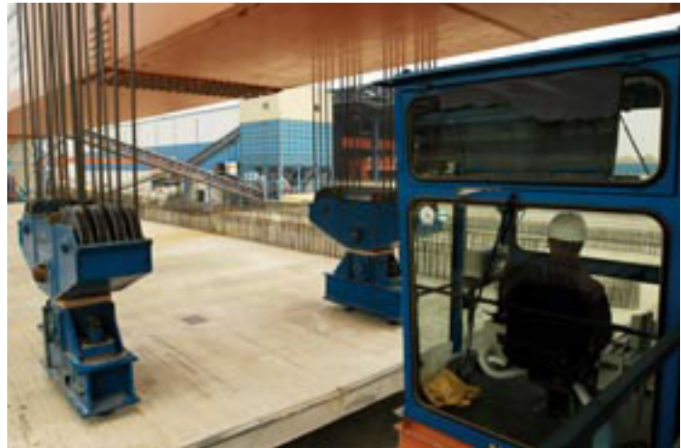
11 Huge beams. Each of the 602 box girders weigh up to 740 tonnes!
