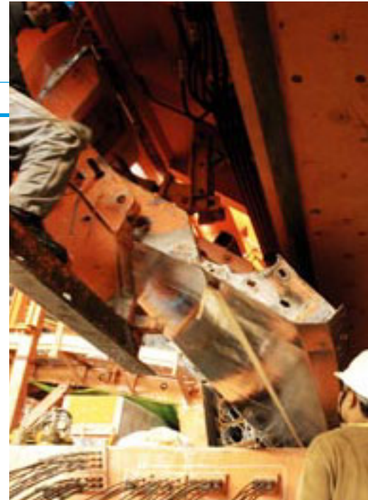
5 Truss launching beam. This 40m long beam is supporting the 30m long inner formwork. On both sides of the beam can be seen the bottom part of the inner formwork. In the foreground, steel bulkhead and coupling strands.
