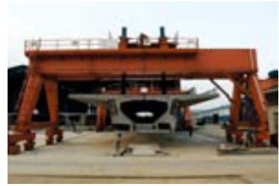
10 Storage. The heavy lifting gantry transfers the box girder to the storage yard.
