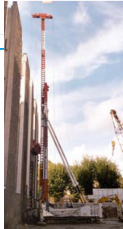
Driving supporting piles
