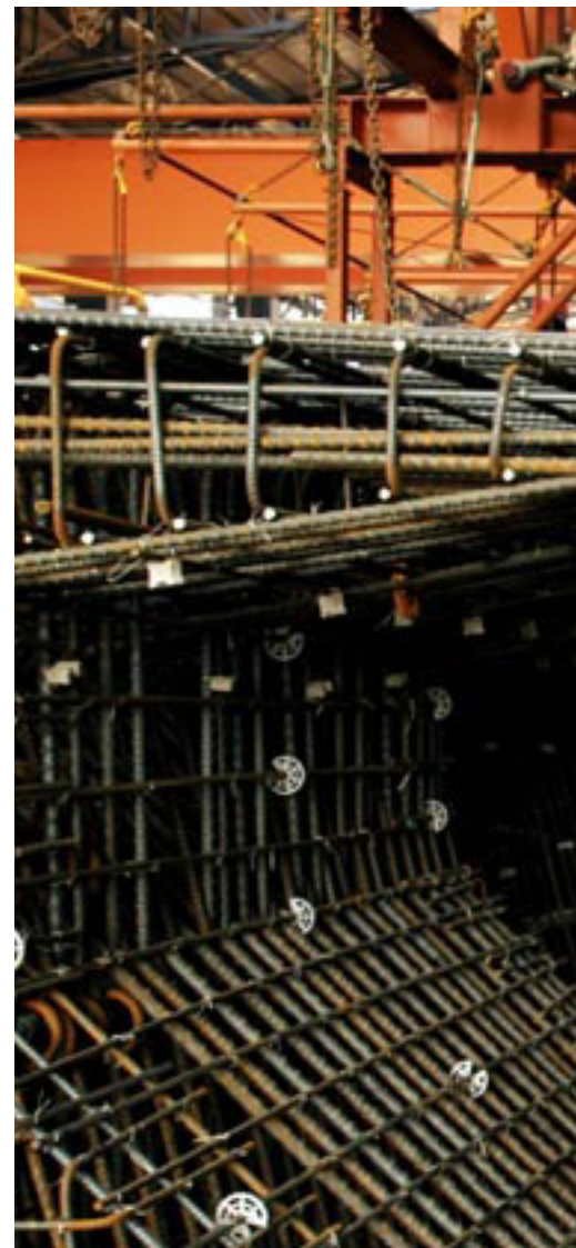
3 Cleaning of external and bottom formwork. Formoil is applied already. In the front left and right side, connected to the bottom form panel is a recess plate with 4 corrugated steel ducts which will form a recess for the dowels of the bridge bearing. On the left side, rebar concrete spacers have already been placed on top of the bearing recess plate and some spacers are now going to be place on the right side.
