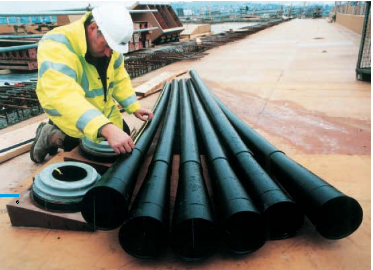
Extralong CS trumpets on Medway bridge deck
