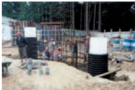
Assembly of a primary panel (two DSEI tube joints)
