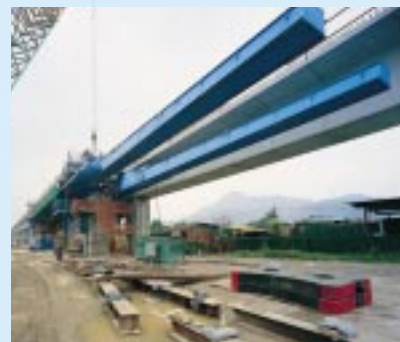
Span-by-span construction using under box girder for erection of multiple parallel decks
