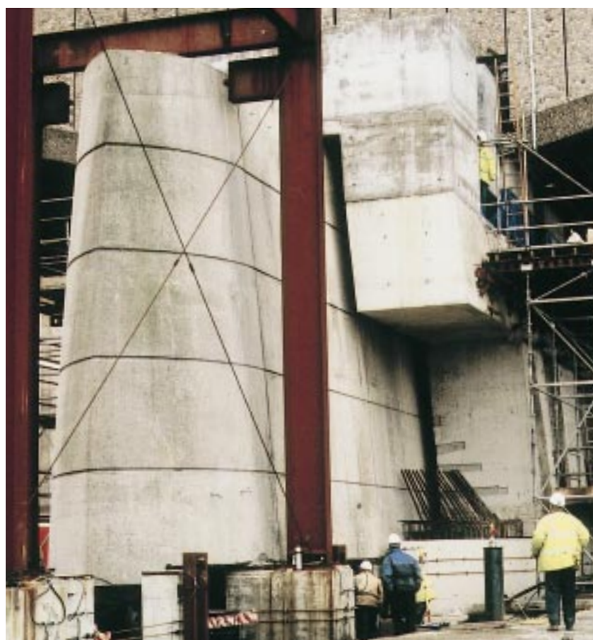
Slide out of main pier shafts
