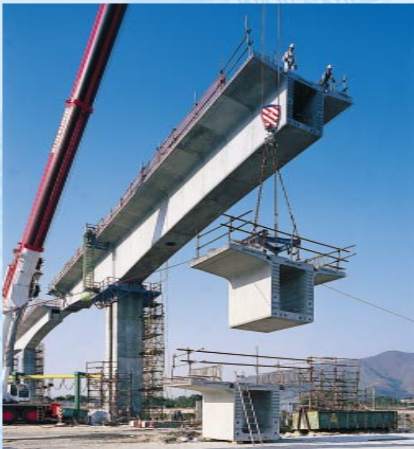
Long span continuous balanced cantilever construction utilising cranes for segment erection.
