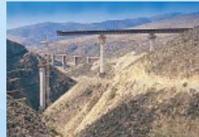
Located 310 km north of Santiago, the Amolanas viaduct is the first launched bridge structure in Chile.
