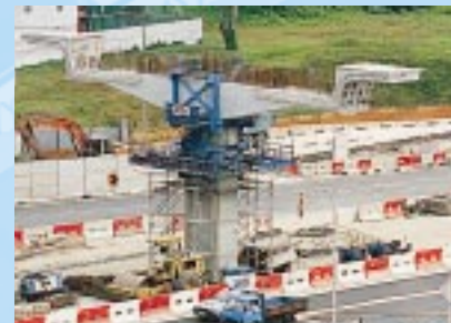
Pre-cast crosshead with support frame and pier corbels. Piers corbels are hydraulically equipped to adjust the crosshead monolithic to the pier.
