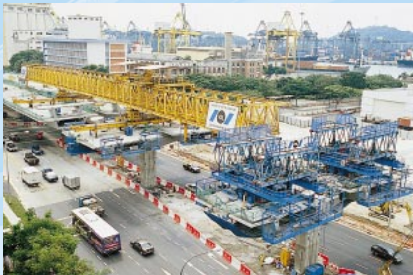
Fore-ground: steel work for the erection of the first pair of segments. Back-ground: gantry for the erection of remaining segments.
