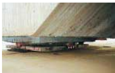
Pot bearing for incremental bridge launching
