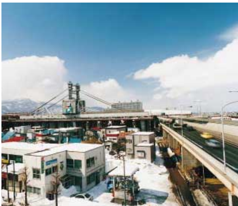
Launching of the bridge girders
