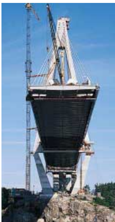
A strand-by-strand installation method
