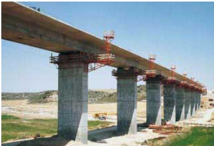
Overall view of High Speed Train viaduct
