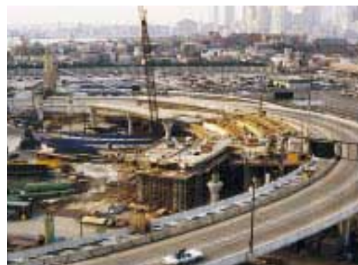
Logan Airport I-90 interchange under construction
