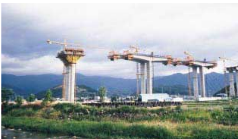
Ku Ryang Chon Free Cantilever Bridge
