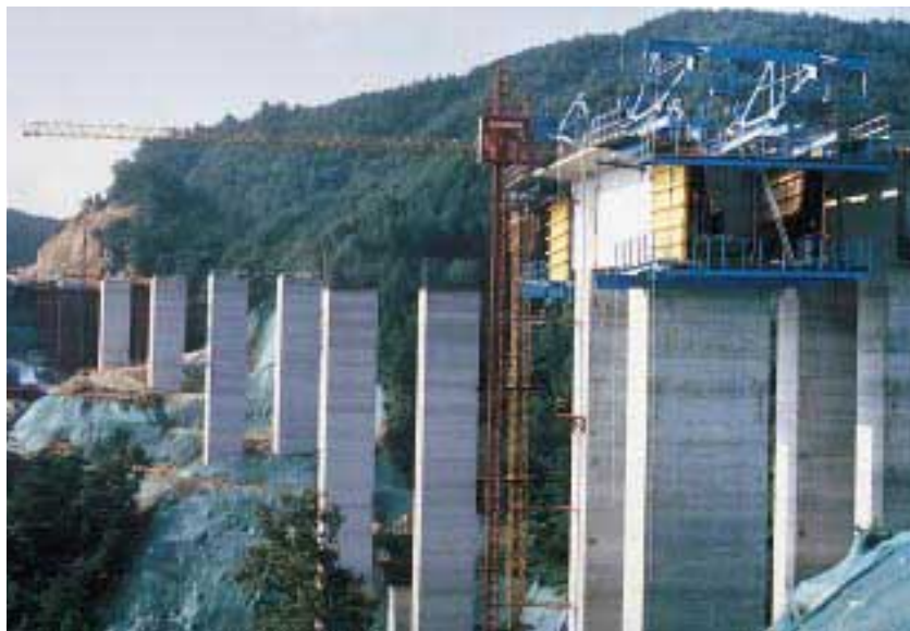
Sungsan Bridge project under construction
