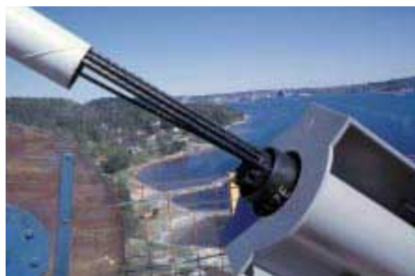
A strand-by-strand installation method
