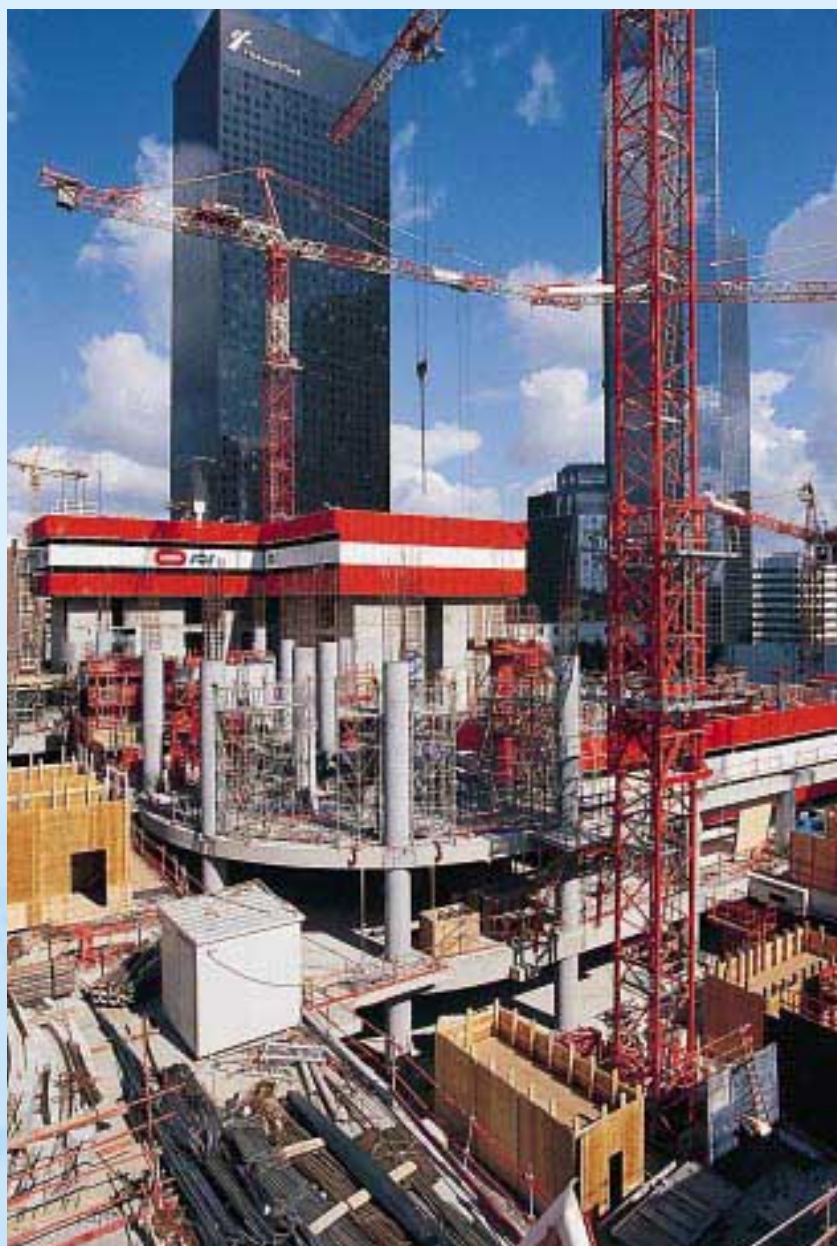
A four-day per-level cycle was achieved using VSL Climbfarm.
