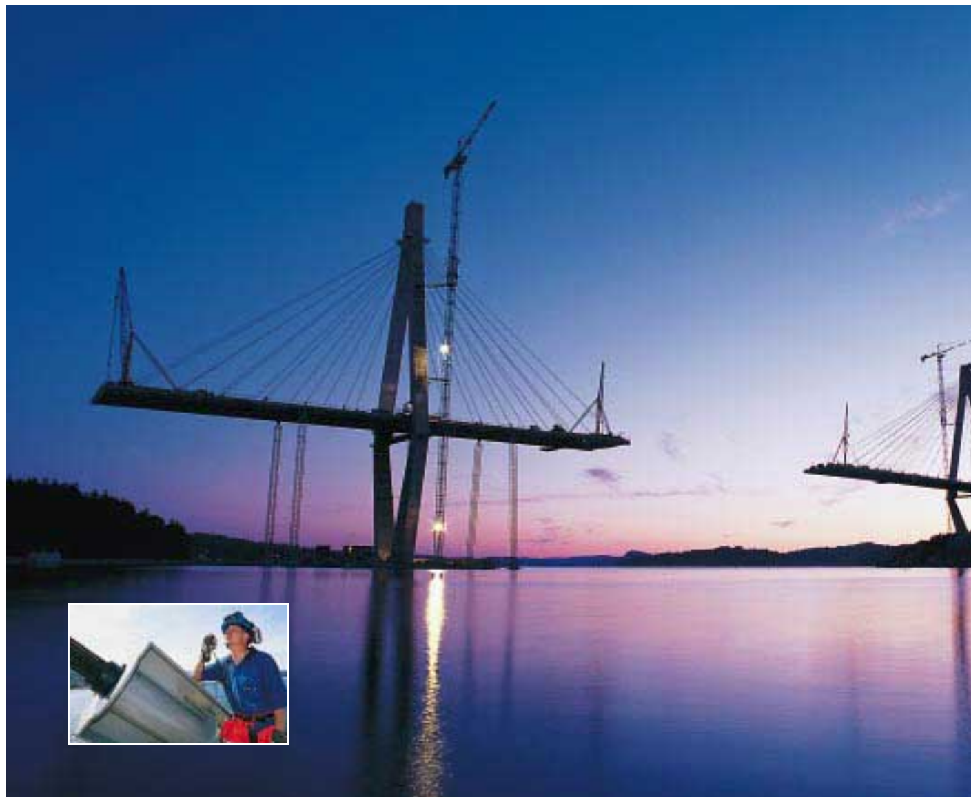
Erection of 120 stay cables (22 to 77 strands) for the Uddevalla Cable-Stayed Bridge
