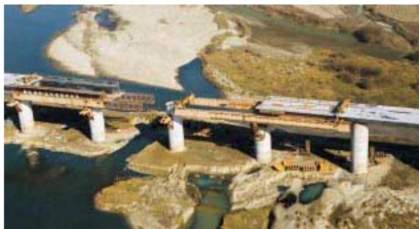
High Speed Rail Section 5-2 constructed with movable scaffolding
