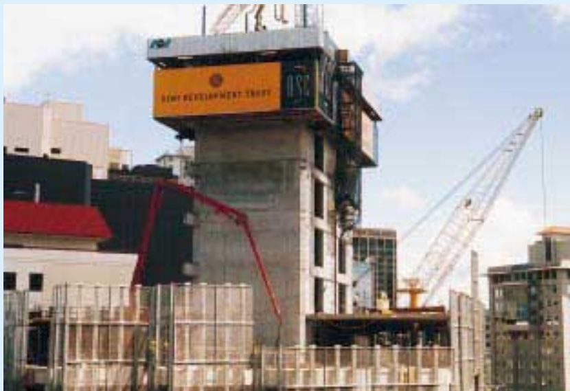
VSL Climbfloor in progress on The Royal Sun Alliance Centre
