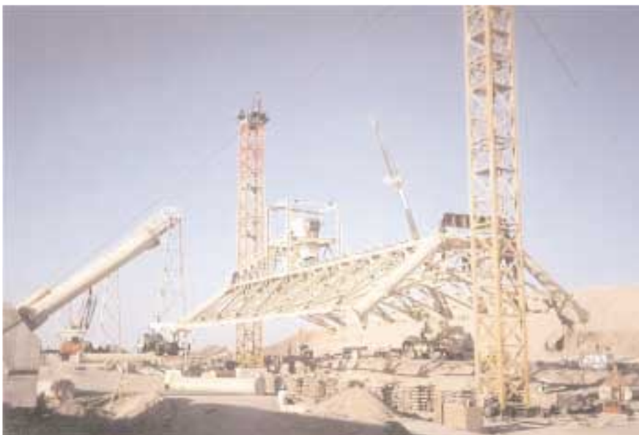
Maria Elena project second lift
