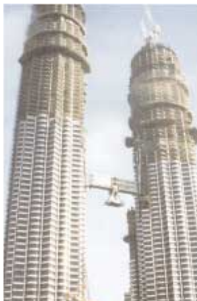
Lifting of the skybridge to link the two Petronas Towers on level 170 m
