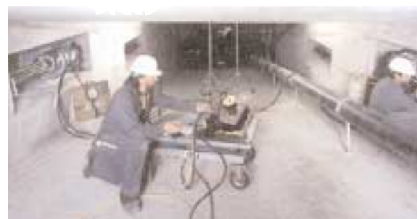
Simultaneous post-tensioning in progress
