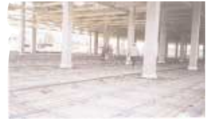
Bayer Plant PT ground slab under construction
