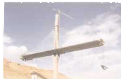
Construction of bridge deck, located 80 m above ground level
