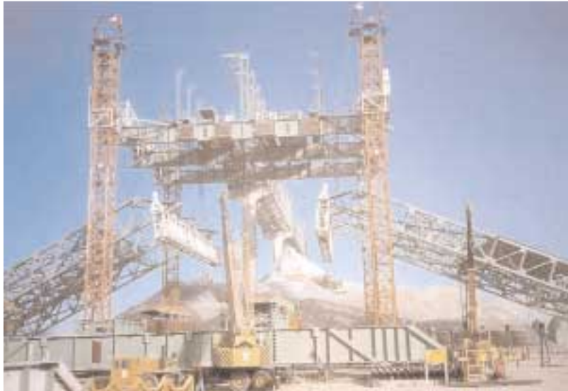
20,000-m 2 steel roof structure, weighing 4,200 t. For erection using the lifting method, the steel roof structure was divided into 8 sections.
