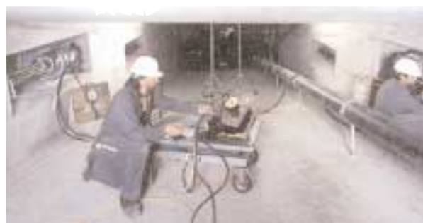
Simultaneous post-tensioning in progress
