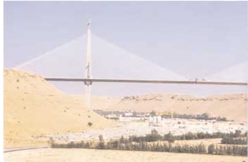
View of the 763-m long cable-stayed bridge crossing the Wadi Leban valley
