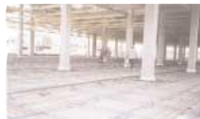
Bayer Plant PT ground slab under construction
