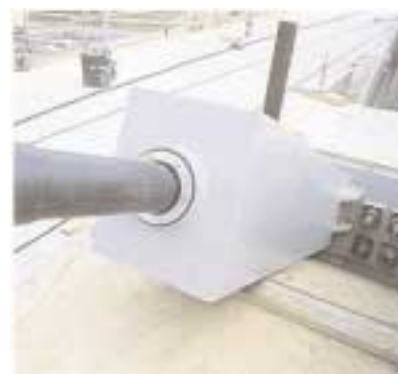
Cables anchored above the deck
