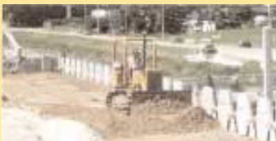
5 • Placing and compacting the backfill
