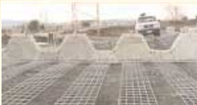
4 • Placing the reinforcing mesh
