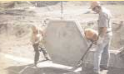
3 • Installing the panels one-by-one
