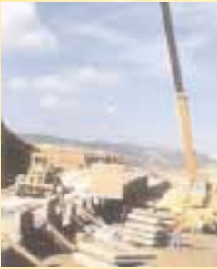
1 • Precasting the panels on site or in a precast yard
