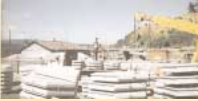
1 • Precasting the panels on site or in a precast yard
