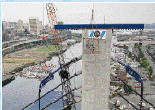
▲ installation of the stays
