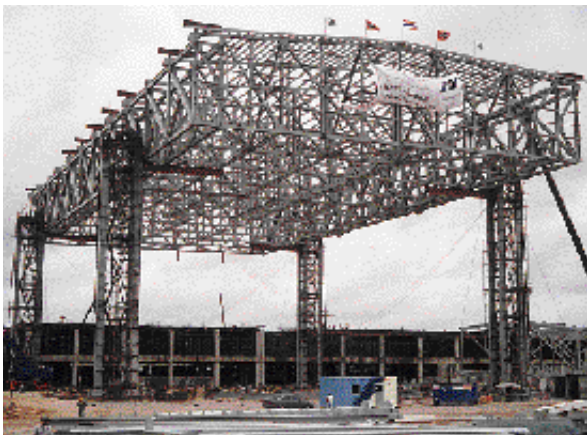
Lifting of the central element weighing 1,200 t and measuring 45 m x 99 m
