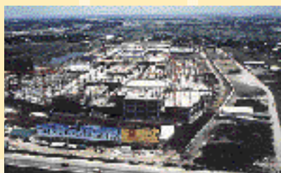
VSL systems are most suitable for commercial shopping centres where large column-free areas are needed. Above is the Fashion Island shopping center in Bangkok where VSL installed 220,000 m 2 of post-tensioned slab
