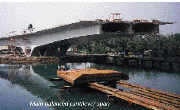
The piers are monolithic and include three V-shaped inclined supports and the pier head segment
