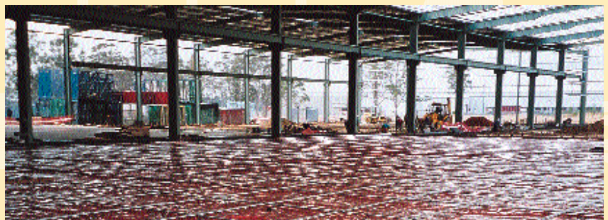
VSL system is suitable for slab-on-ground applications. In the Pilkington glass plant in Australia, VSL installed 22,000 m 2 of crack free, durable PT ground slab.
