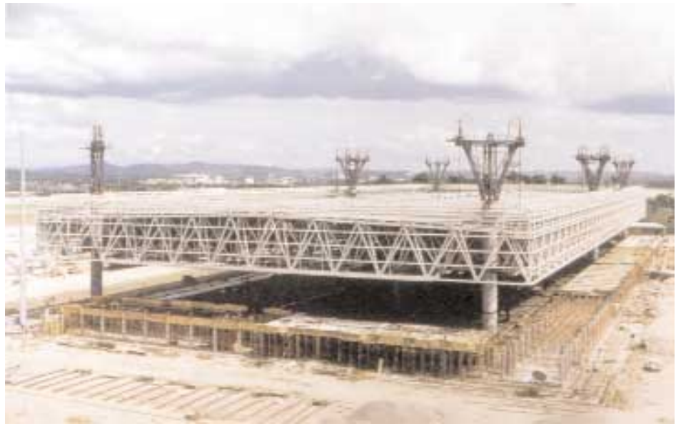
The hangar roof during lifting and a close-up of a column with 4 strand lifting units
