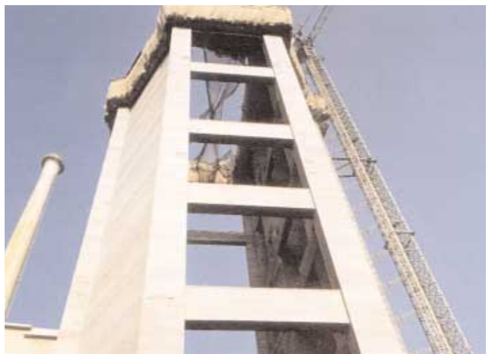
The Unicem furnace tower near Bari, Italy
