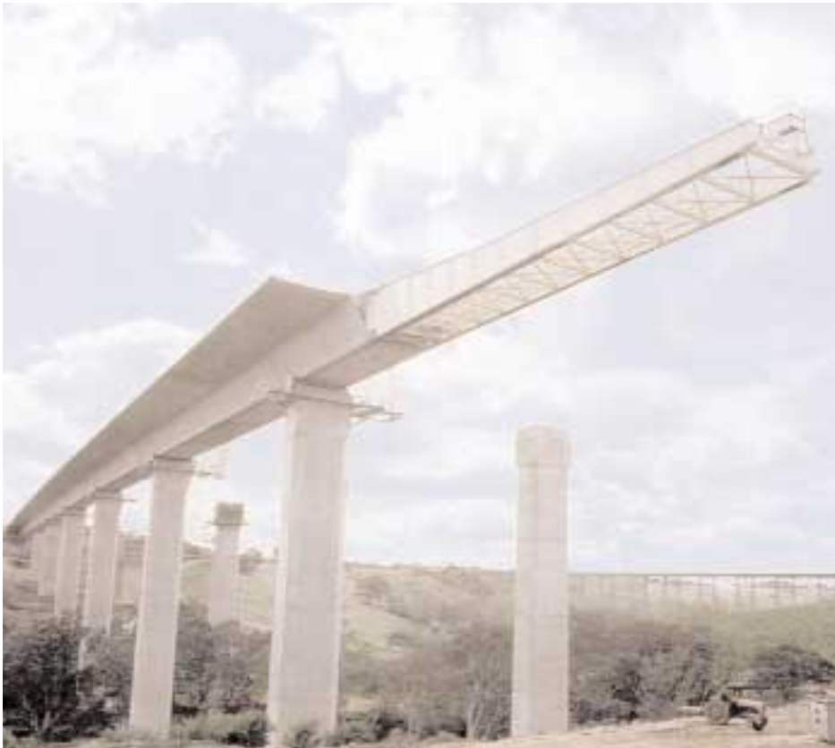
Western carriageway during launching
