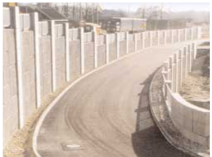
Attractive retained earth walls, France
