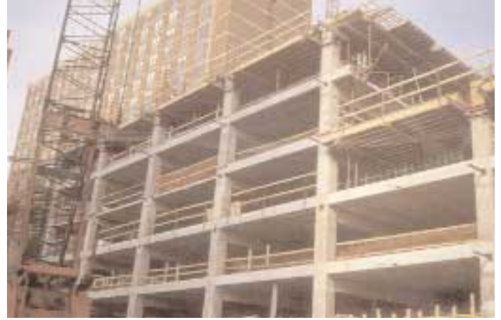
Overall View – Hahnemann parking garage under construction
