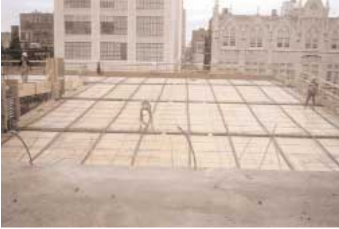
Installation of PT-PLUS flat duct
