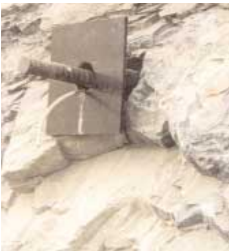
Electrically isolated passive bar anchor
