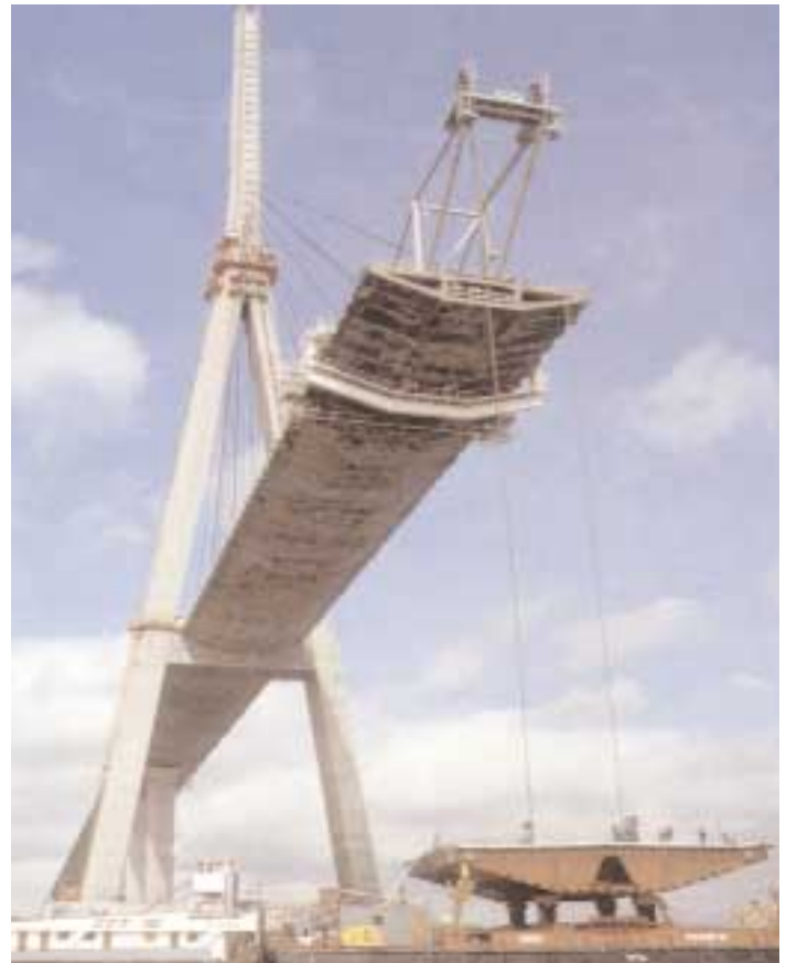
Segment erection Normandy Bridge
