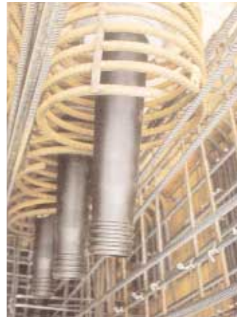
CS anchorages installed
