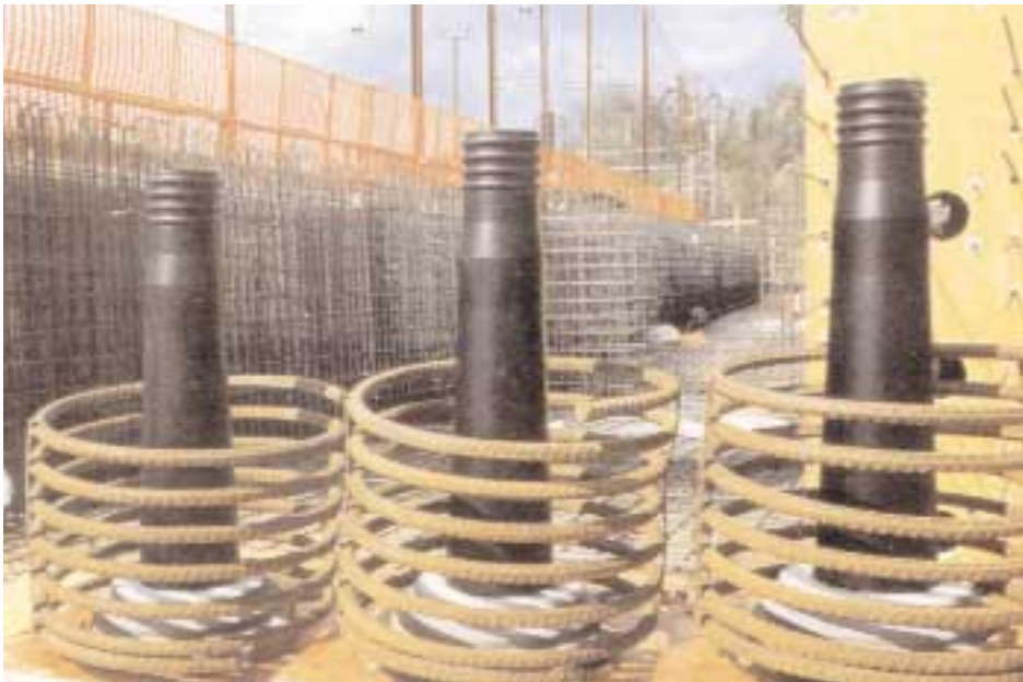
The new Aare railway bridge, Brugg, Switzerland
