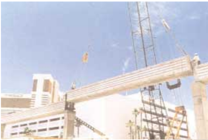
Placement of precast guideway segment
