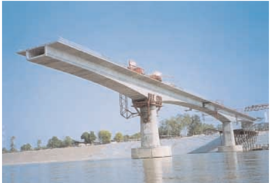
Balanced cantilever construction at Mekong River Bridge
