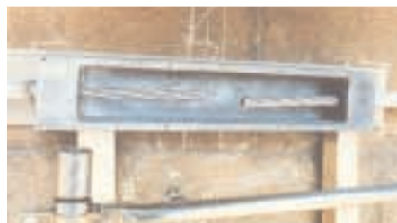
Circumferential prestressing single strand anchorage body
