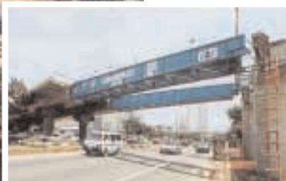
Overall bridge with casting yard in the background, and launching nose position before reaching the pier, spanning the main street of Sudirman
