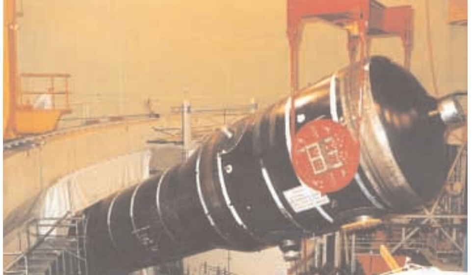
Exchange of steam generator
