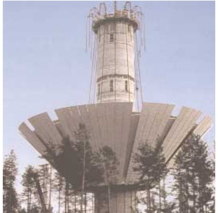
VSL heavy lifting serves the needs of this water tower construction.
