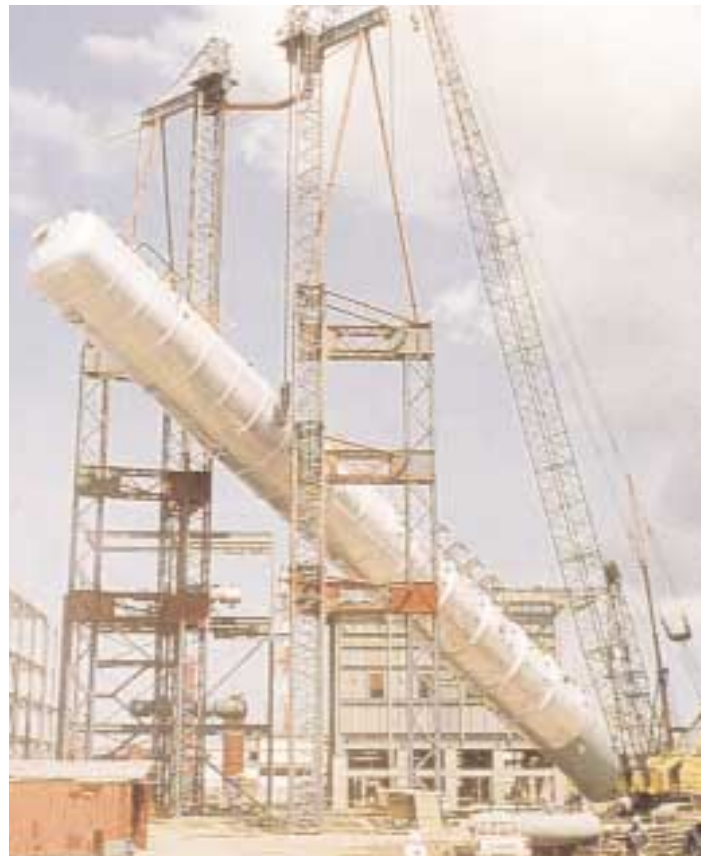
VSL Lifting Towers without guy wires solve Trinidad Lifting problem.
