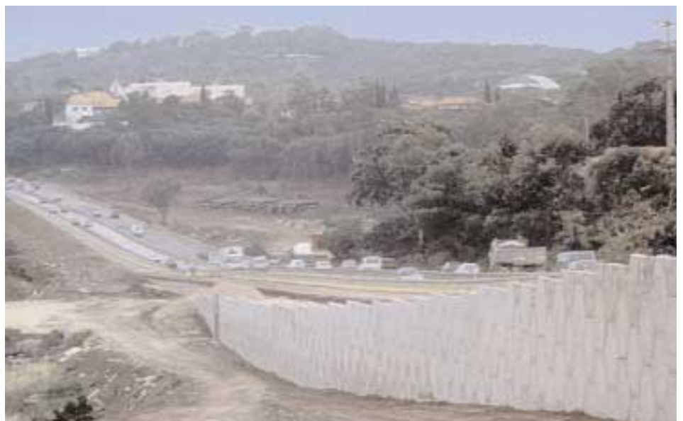
Retained Earth panels support embankment of a widened highway in Portugal.
