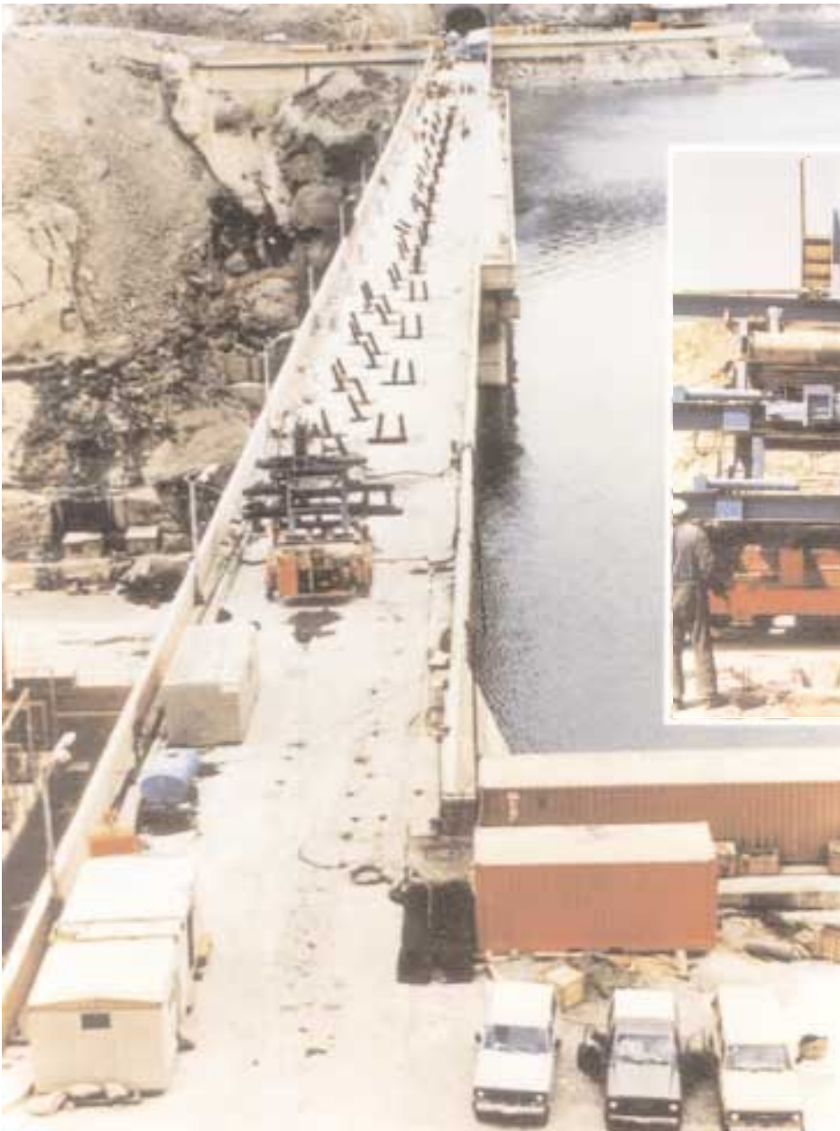
A total of 234 permanent rock anchors tie the cracked upper section of the dam to the stable lower concrete
