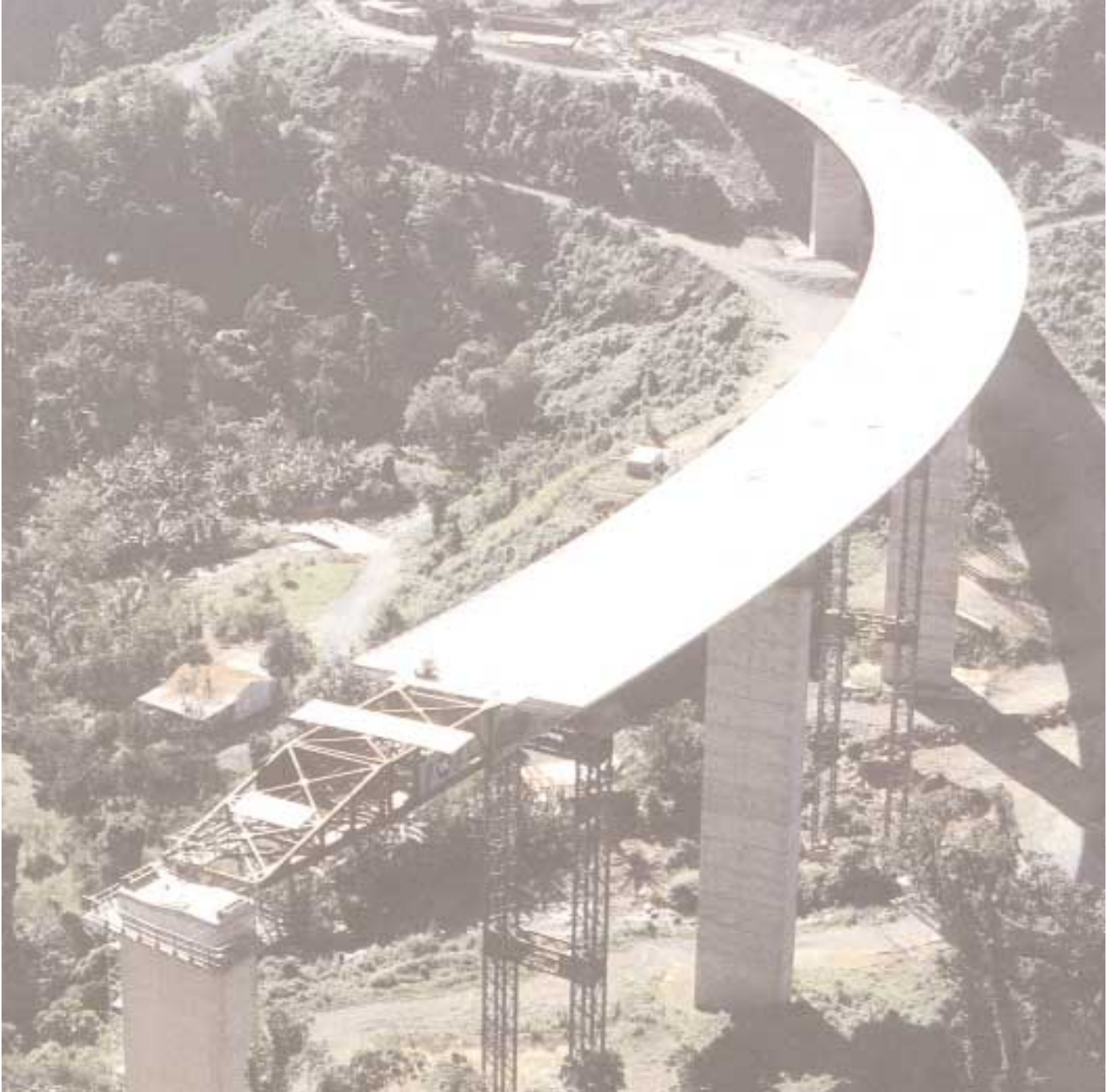
The Caguanas River Bridge, built by the VSL Incremental Launching Method.
