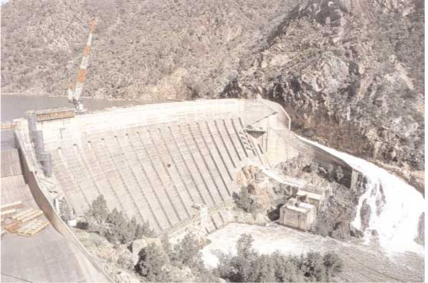
Work has begun to strengthen Burrinjuck Dam.
