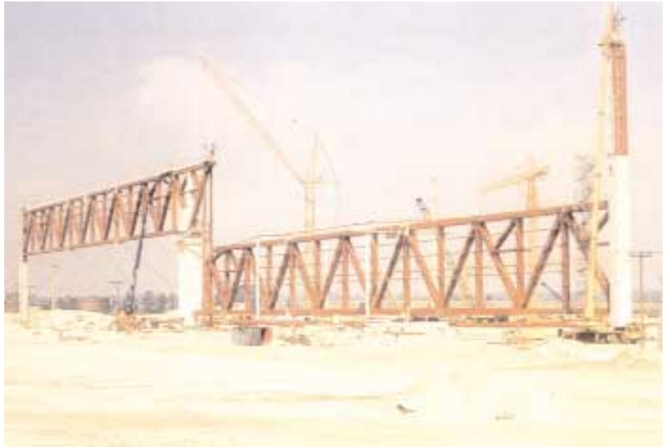
Lifting of 150m long hangar doorway truss
