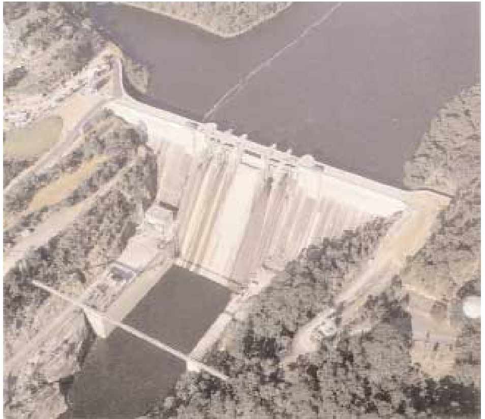
The raised and strengthened Warragamba Dam.
