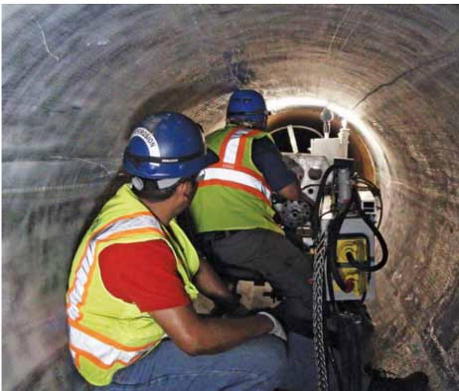
← The hybrid FRP system was successfully installed and restored full functional capacity of MDWASD's high-risk pipeline segments by increasing the structural capacity.
