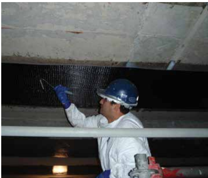
Installation of the FRP Composite Strengthening System.
