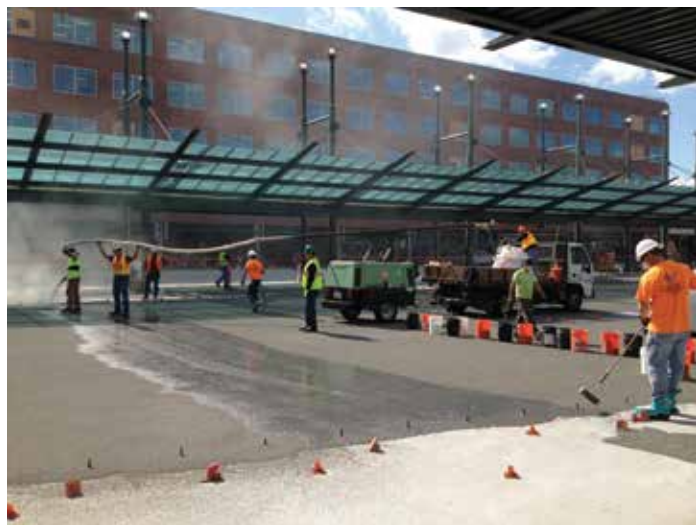
Crews apply a traffic-bearing coating in the public transportation area.
