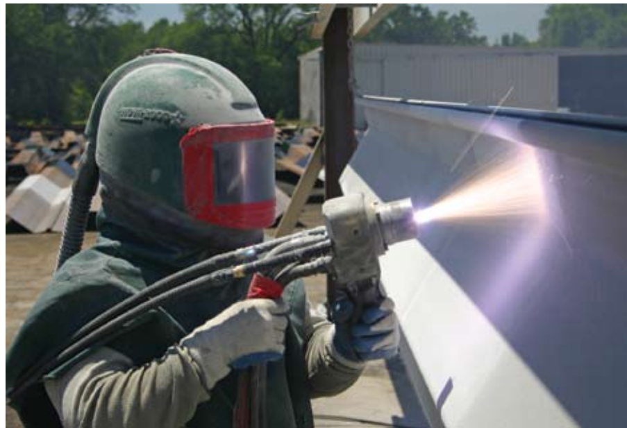
Metallizing for corrosion protection of steel using wire arc system
