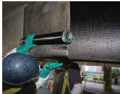
FRP fabric is easily tailored to fit any geometry, including 'U' wrapping around beams.
