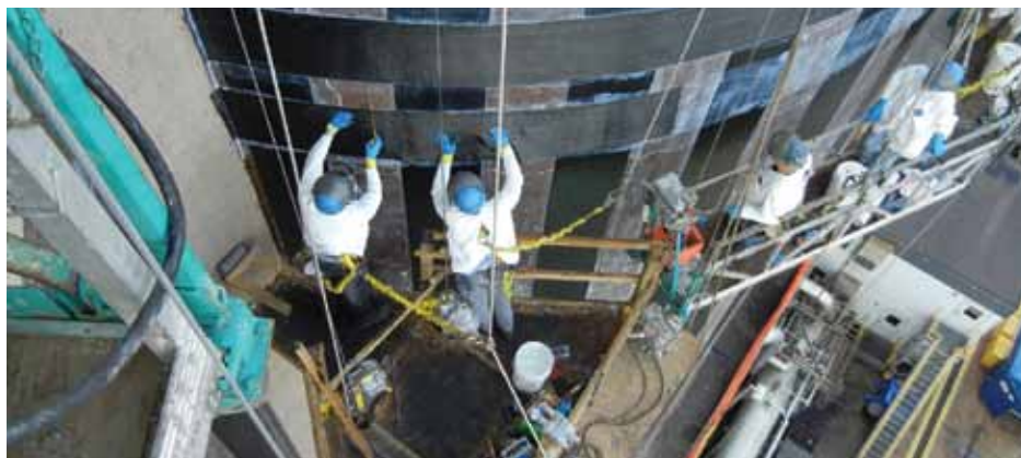
Installation of CFRP on an industrial silo.
