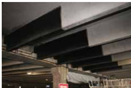
CFRP reinforcement on parking garage beams.
