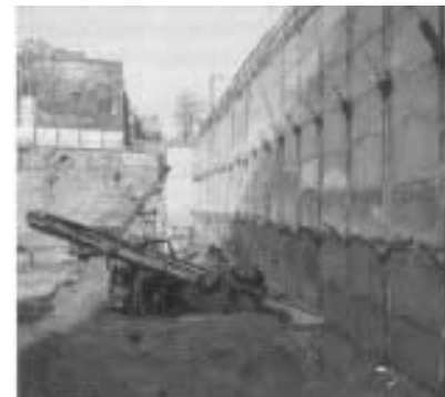
Fig. 41: Anchor work
