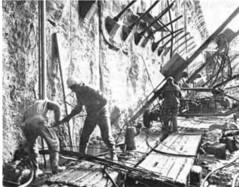
Fig. 48: Execution of the anchor works
