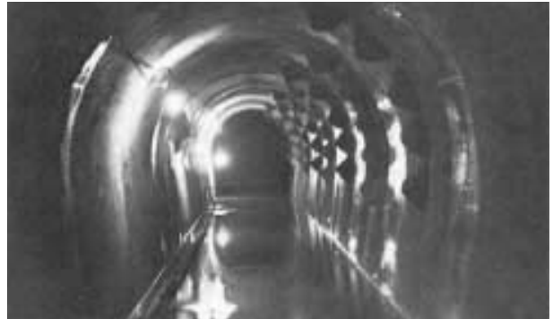
Fig. 17: Drainage tunnel with anchorage blocks
