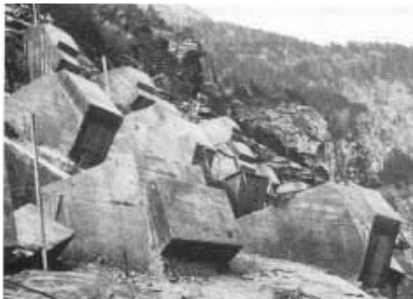
Fig. 6: Anchorage blocks of 1400 kN-anchors
