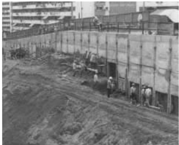
Fig. 45: Construction of Berlin wall
