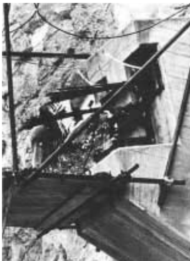
Fig. 73 Anchor work on an upper foundation
