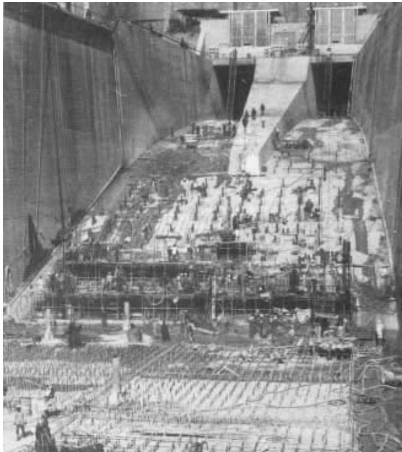
Fig. 57: The stilling basin during anchor work
