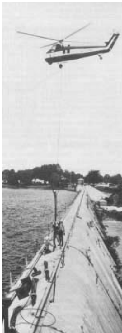
Fig. 83: Positioning of the anchors
