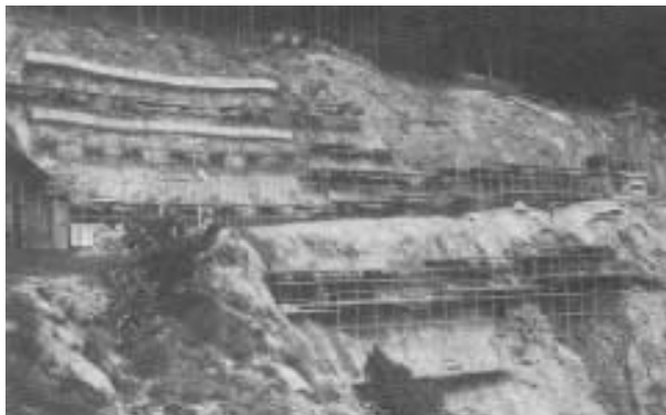
Fig. 12: Overall view of the slope during drilling operations in the middle section
