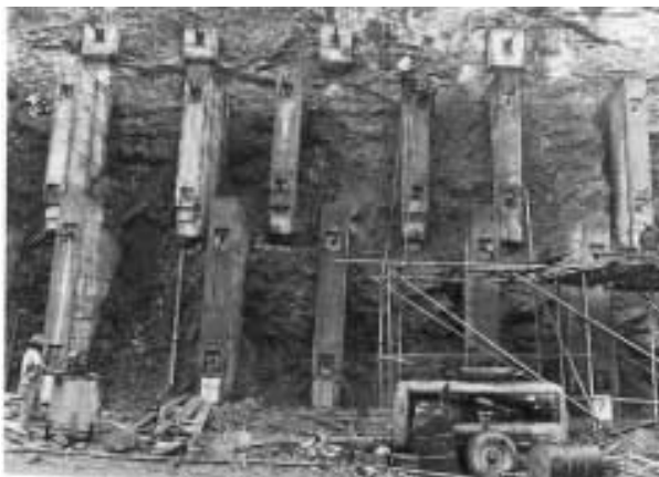
Fig. 27: Anchored concrete tie-beams
