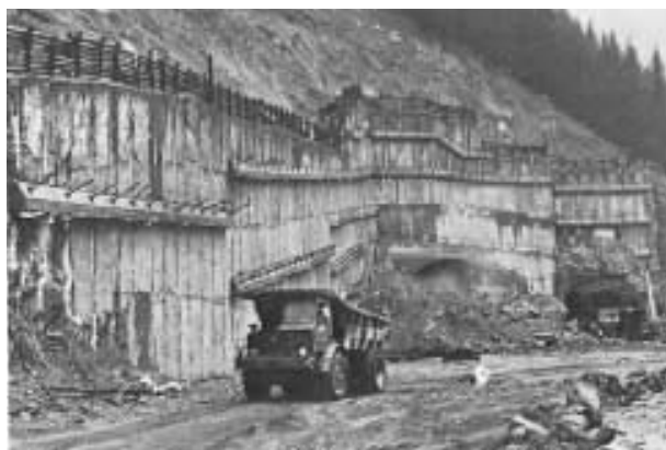
Fig. 33: View of the anchored pile wall
