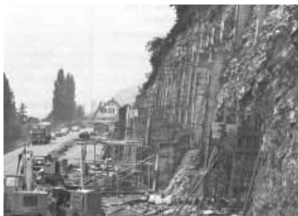
Fig. 29: Construction of staggered wall
