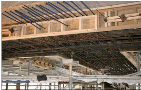
Strengthening Solutions- External PT and Enlargement
