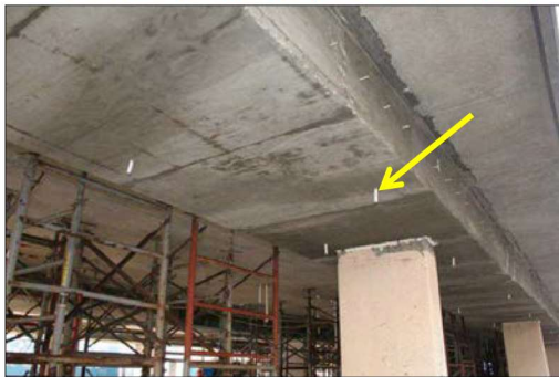
Strengthening Solutions- External PT and Enlargement Vents in F&P formwork for placement confirmation
