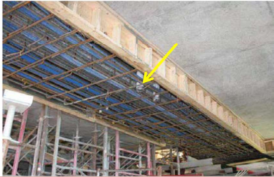
Strengthening Solutions- External PT and Enlargement
