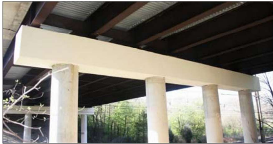
Completed Bridge Pier - FRP Strengthening
