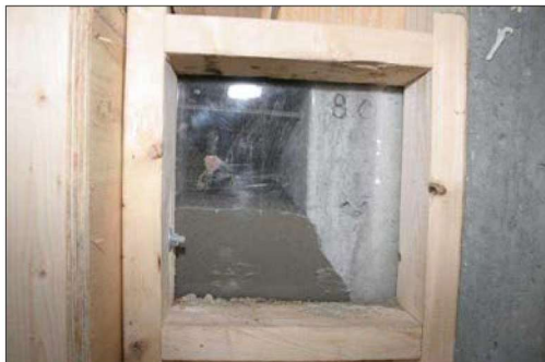
Strengthening Solutions- External PT and Enlargement Window in F&P formwork for placement confirmation
