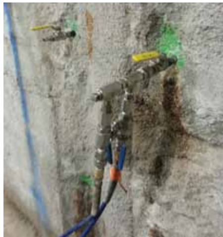
To achieve the right mixing ratio of water to grout, a multi-ratio pump should be used.
