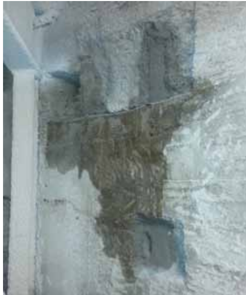
Monolithic concrete with a compressive strength in excess of 3500 PSI is watertight, except at any irregularities.
