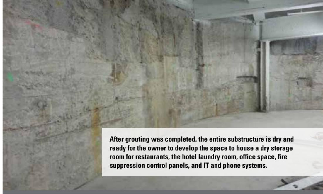
**After grouting was completed, the entire substructure is dry and ready for the owner to develop the space to house a dry storage room for restaurants, the hotel laundry room, office space, fire suppression control panels, and IT and phone systems.**
