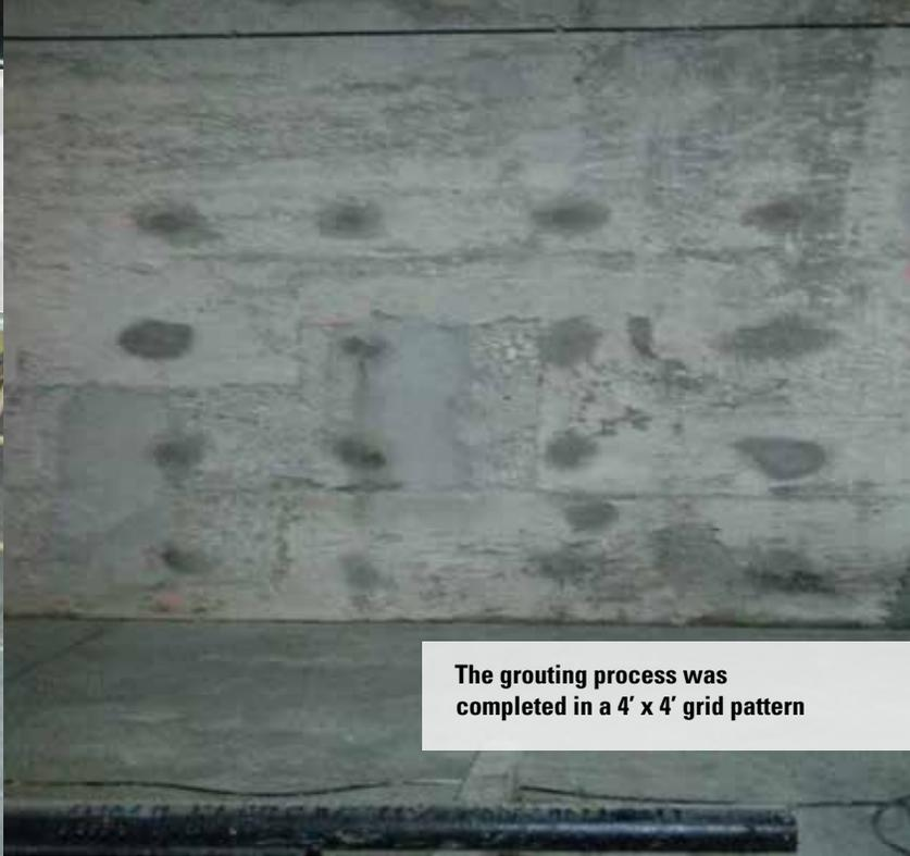
**The grouting process was completed in a 4' x 4' grid pattern**
