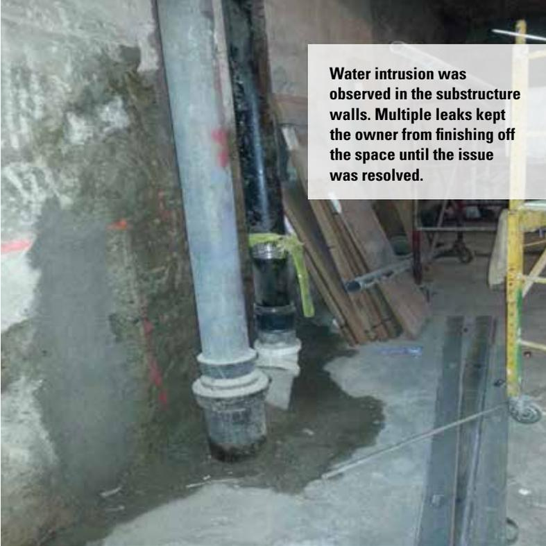
**Water intrusion was observed in the substructure walls. Multiple leaks kept the owner from finishing off the space until the issue was resolved.**
